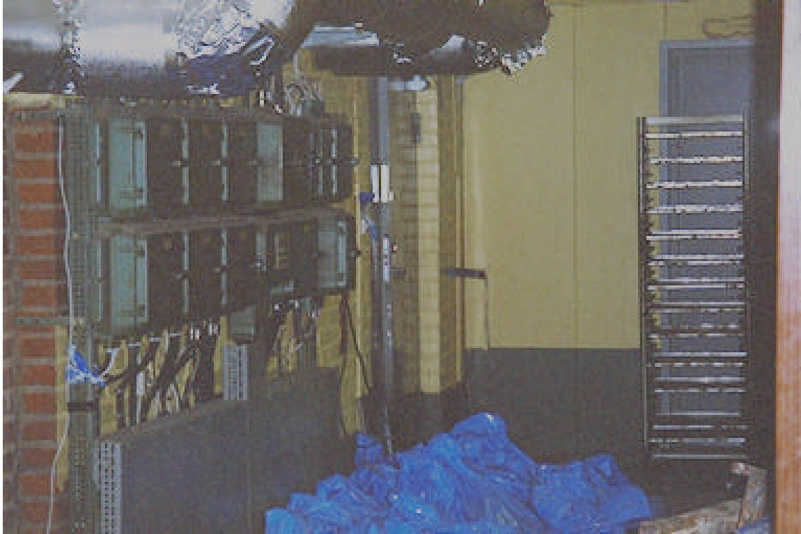
Photo No. 4 – The door at the bottom of the southeast exit from the hall discharged into a common corridor area. (NFPA)
