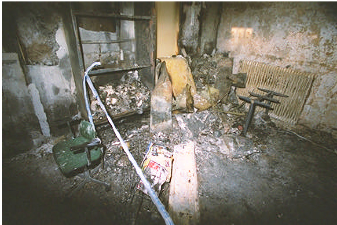
Photo No. 12 – The furnishings in the Main hall comprised mainly of combustible materials over metal frames.
