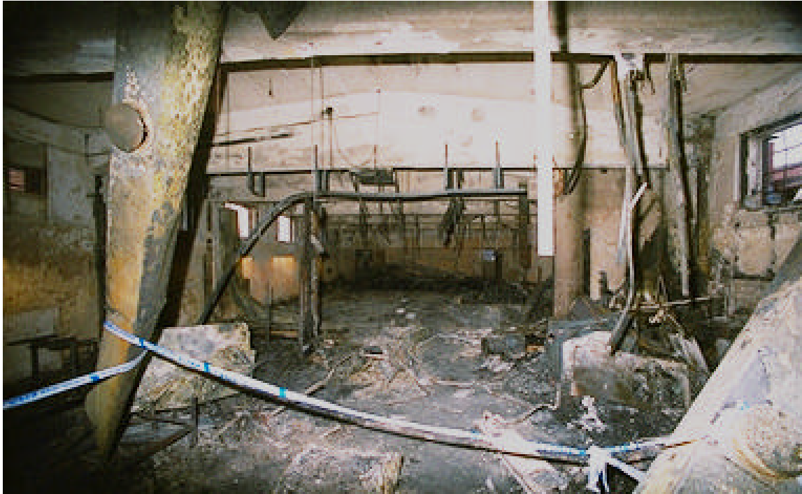
Photo No. 10 – This is a view of the interior of the main hall from the entrance looking towards the stage. (Note: None of the contents had been removed from the area when this photo was taken.)
