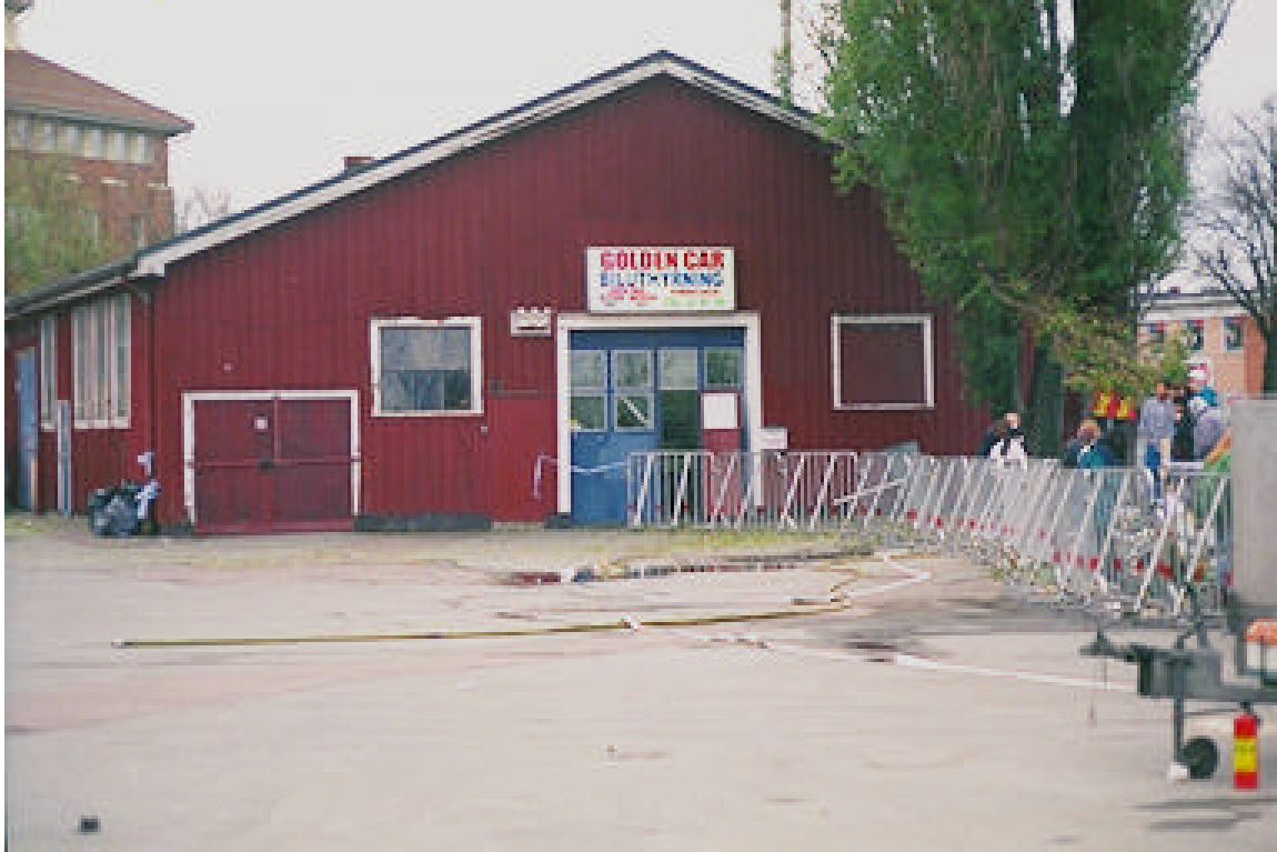
Photo No. 8 – This adjacent garage was forced open and used as a triage center for the injured victims. (NFPA)
