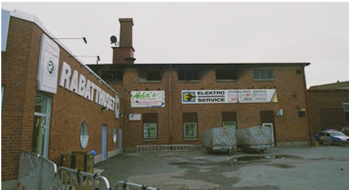
Photo No. 7 – Exterior view of building showing the windows that had been broken out on the second floor and where occupants jumped to the ground. (NFPA)
