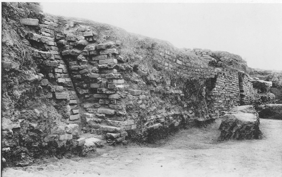
b. The retaining-wall of the Ziggurat platform, showing Kuri-galzu's revetment of the Kudur-Mabuk frontage
