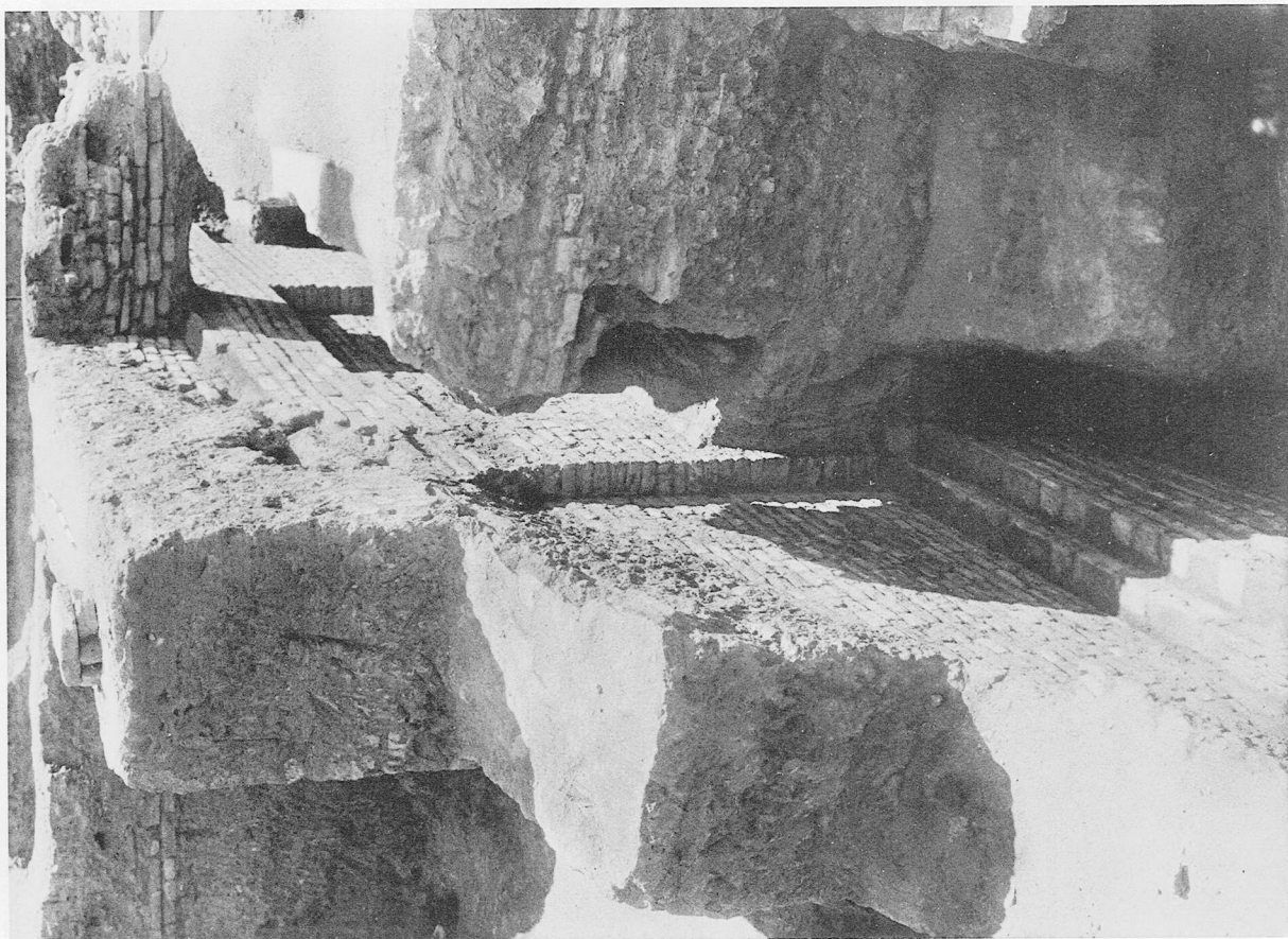
b. View looking SE along the outer (SW) wall of the B range.
