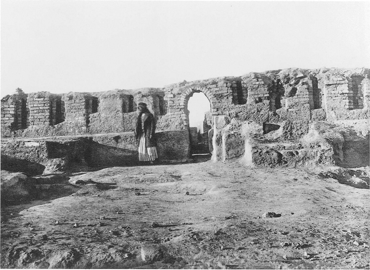
a. The NE side, before the removal of Sin-balaṣu-iqbi's mud-brick additions
