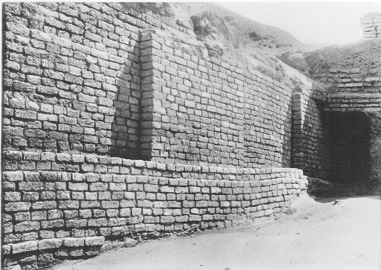
a. The outer face of the butressed wall dividing sections B and C.
