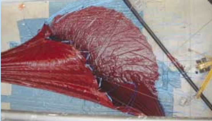
10. Membrane at east end viewed from above prior to erection.
