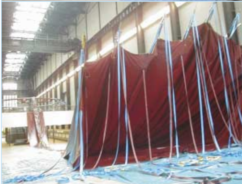
8. Raising membrane at east end.
