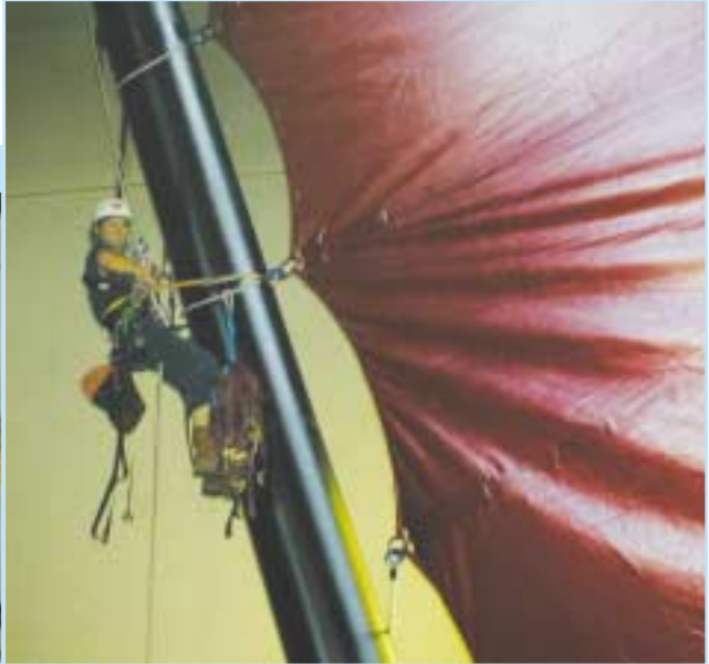
9. Abseiler securing connection
