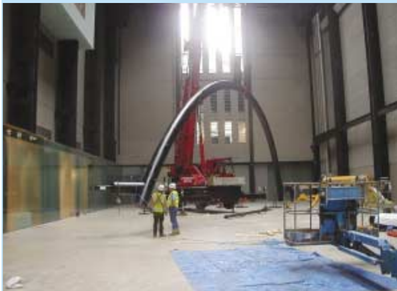
7. Commencing erection of east steel ring.
