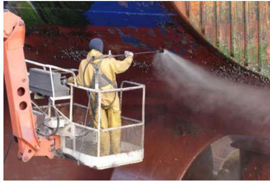
Figure 1: Initial removal of fouling epibiota by water blasting at Tauranga Marina (A) and Lyttelton dry dock (B).
