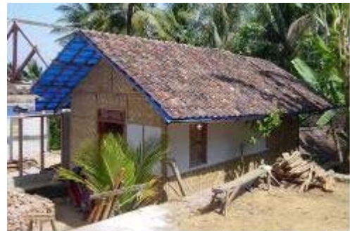
Figure 2: Utilizing Plastic Sheeting in Transition to Permanent Shelter
