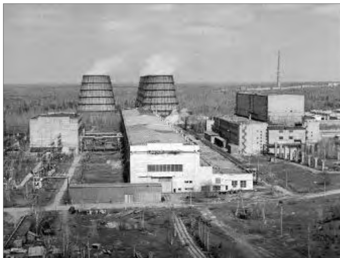
The ADE reactors are perhaps the least safe reactors in operation today.
