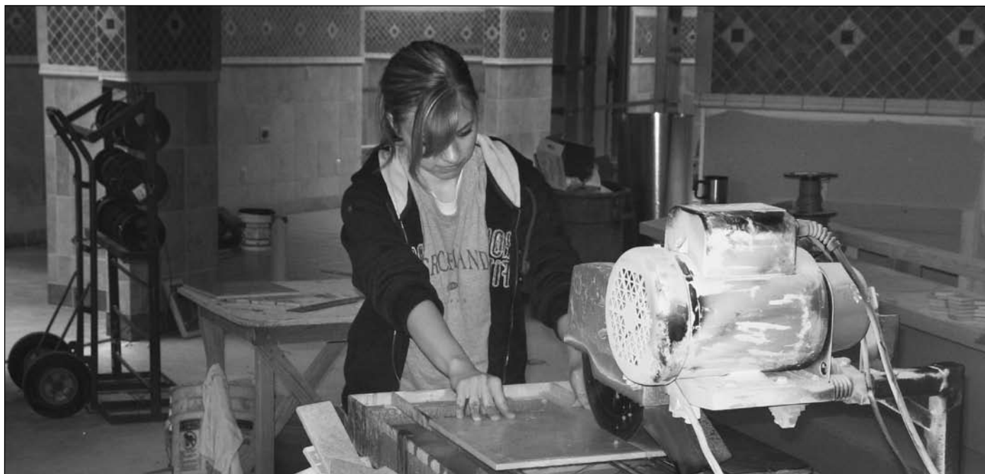
The dining room takes shape as student Stephanie Wiggs cuts a piece of tile to add to the wall.
