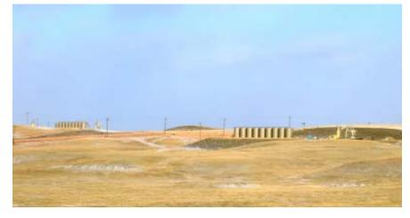
Figure 3. Two oil leases in southern Mountrail County. Photograph taken looking northeast. The wells in this area are on 640-acre spacing, but these two leases are close together because the horizontal leg of the oil well to the left was drilled from southeast to northwest and the horizontal leg of the oil well on the right was drilled just the opposite, from northwest to southeast.
