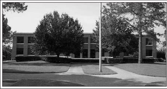
Alvin I. Thomas Administration Building
