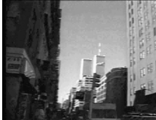
Figure1. Impact of WTC 1, North tower
