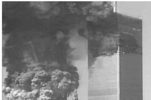
Figure 3. Collapse of the South tower
