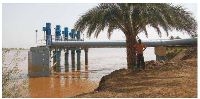
Riverbank erosion removed the supports of this irrigation pump intake system within months of its installation, and threatens to destroy it completely. Without mitigatory measures, the site is not suitable for such a project
