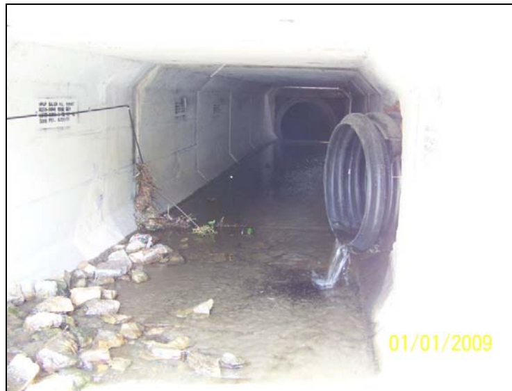
Figure 3. Section culverted underground, Progress Street at Rescue Squad (Source: Parece 2009)
