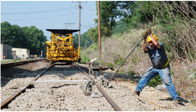
This image shows a track worker conducting much needed maintenance. An NAUG track worker is jacking and leveling the track in preparation for the tamping machine to vibrate and compact the stone ballast around and beneath the wooden crossties.
