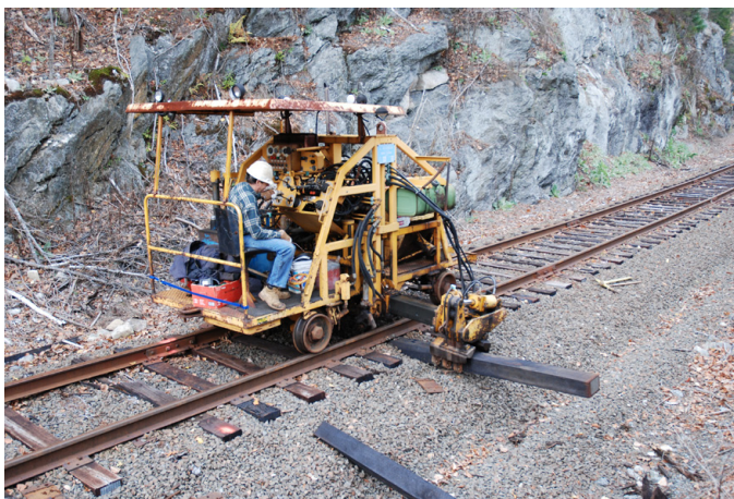
This image shows NAUG crosstie insert machine making repairs.
