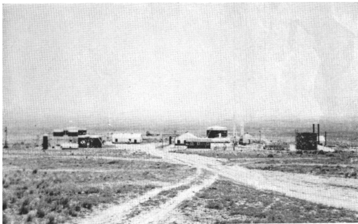
B. Crude-oil stabilization plant and electric light plant of Continental Oil Co., Rattlesnake field. San Juan County.
