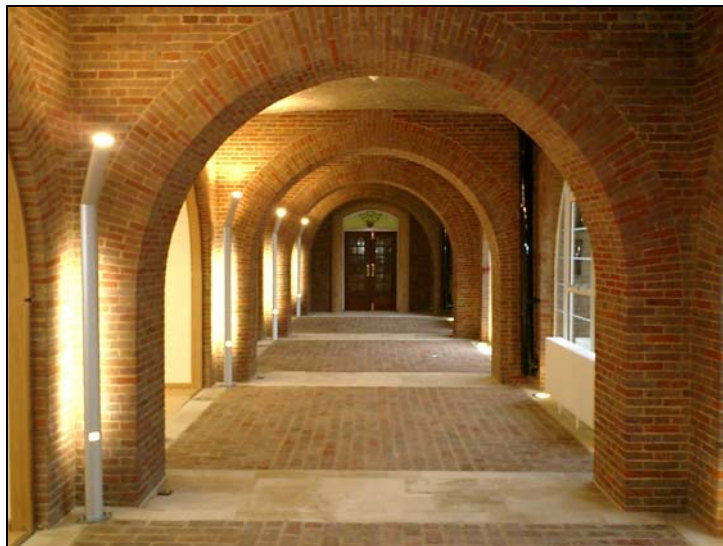
The refurbished Undercroft
