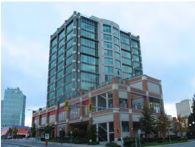
Fig. 1 North-east view of the test-site.
