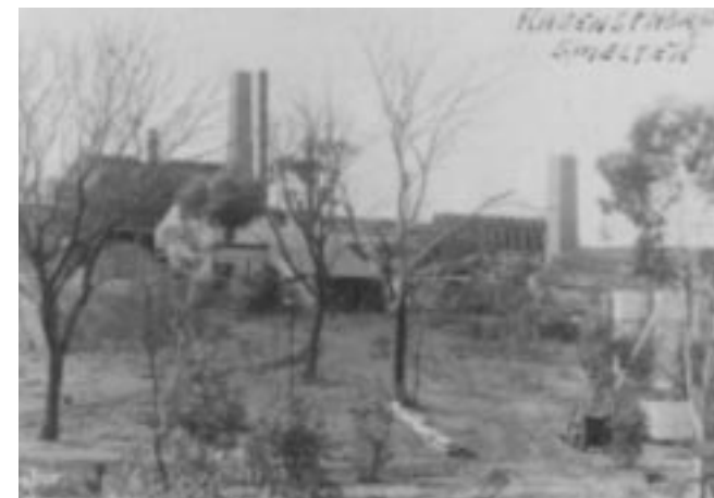
Ravensthorpe Smelter, 1908 (courtesy Ravensthorpe Historical Society).
