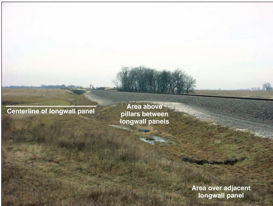
Figure 14 This railroad grade was re-established after longwall coal mine subsidence by increasing the vertical amount of crushed rock (ballast) below rails where longwall panels crossed under the tracks. (Photograph by Dan Barkley.)
