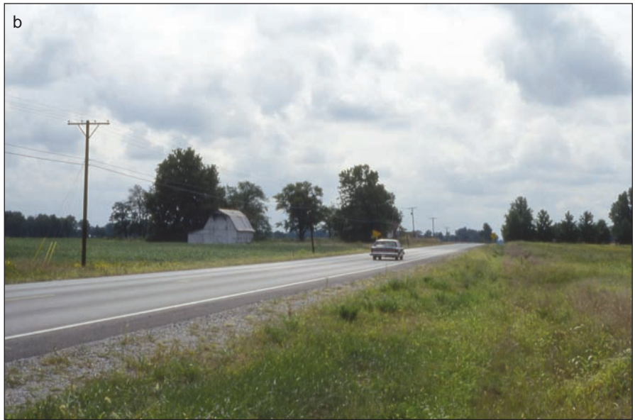
Figure 13 Examples of a road subsided (a) over a longwall panel and (b) repaired.
