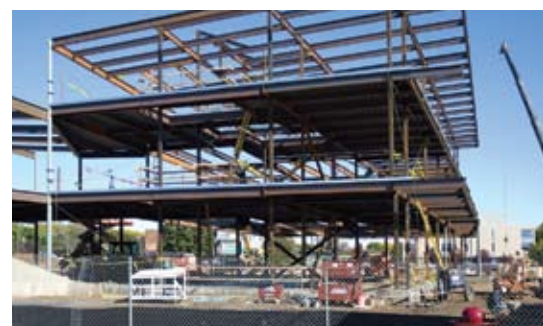
New Business Building
