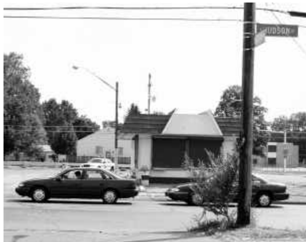
Existing Conditions along Hudson Street.
