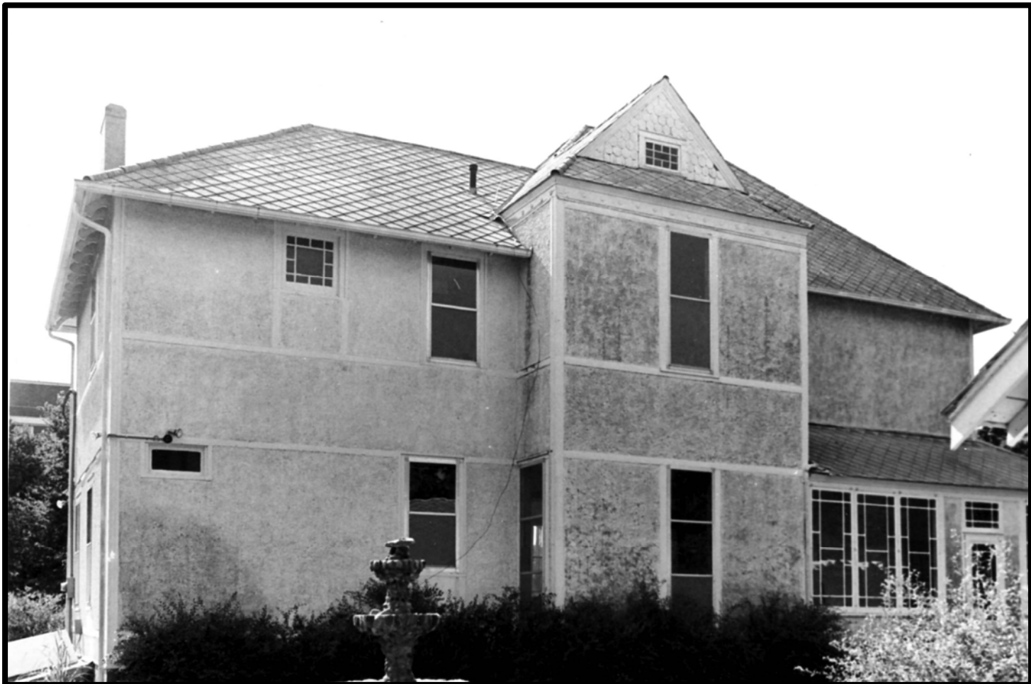
Photo 4 of 7 – E façade. Photo by Janet Jeffries Spencer, 1980, NSHS (8007/41:19)
