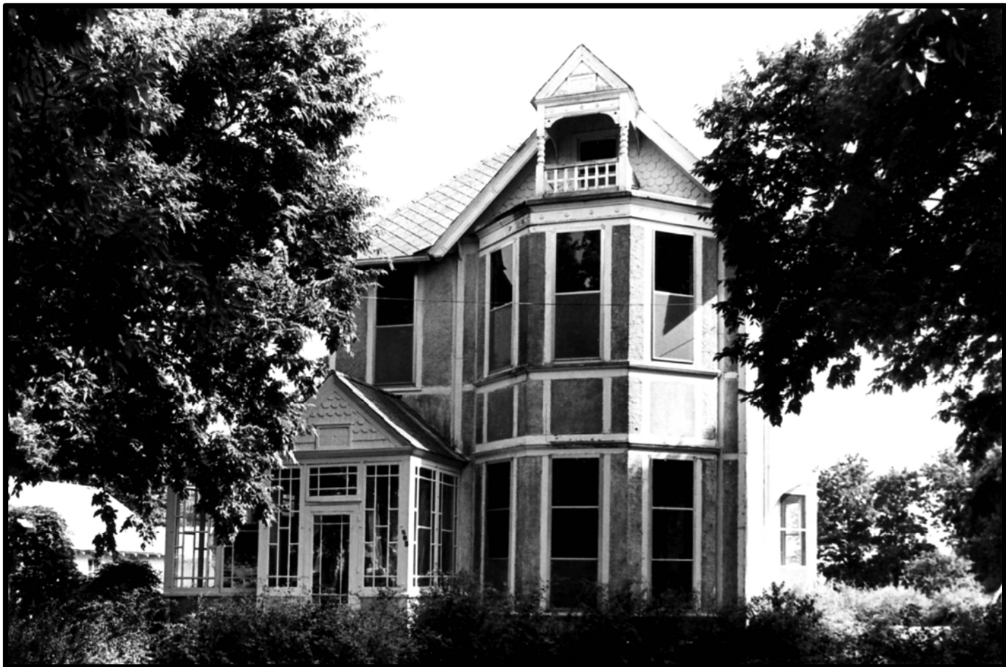
Photo 1 of 7 – N façade. Photo by Janet Jeffries Spencer, 1980, NSHS (8007/41:15)
