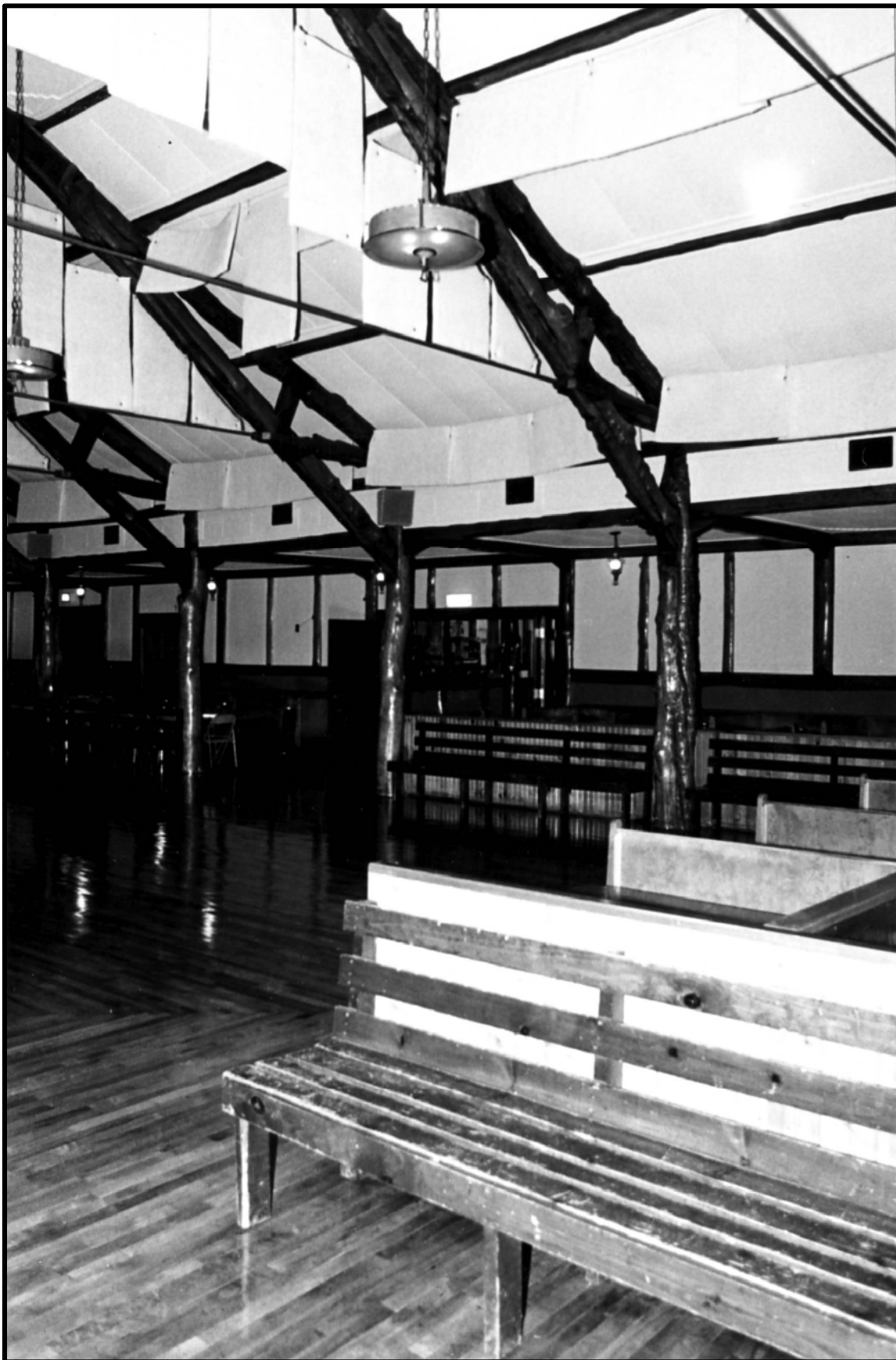
Photo 9 of 10 – view looking west across dance floor toward the bar and lunch room Photo by D. Murphy, NSHS, March 1980 (8003/9:5)
