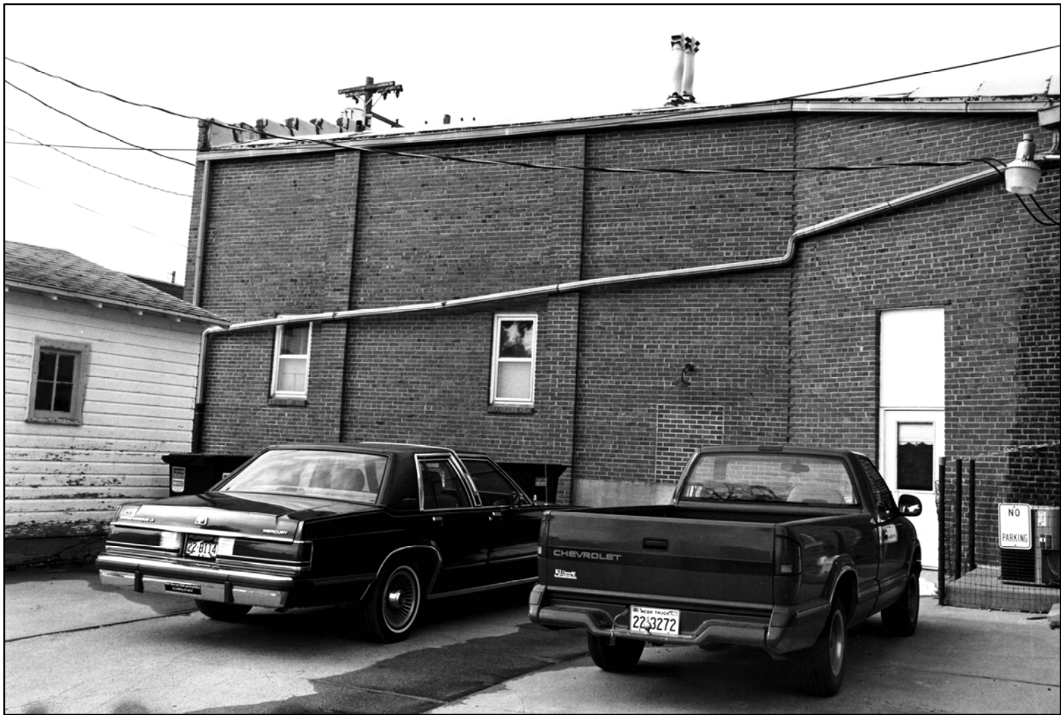
Photo 4 of 4 – view showing south façade Photo by Greg Miller, March 1998, NSHS (9803/1:12)
