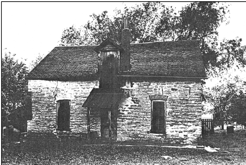
Photo 4 of 17 – House east (rear) façade Photo by D. Murphy, Lincoln, NE, 1975 (DM 7505b:30)
