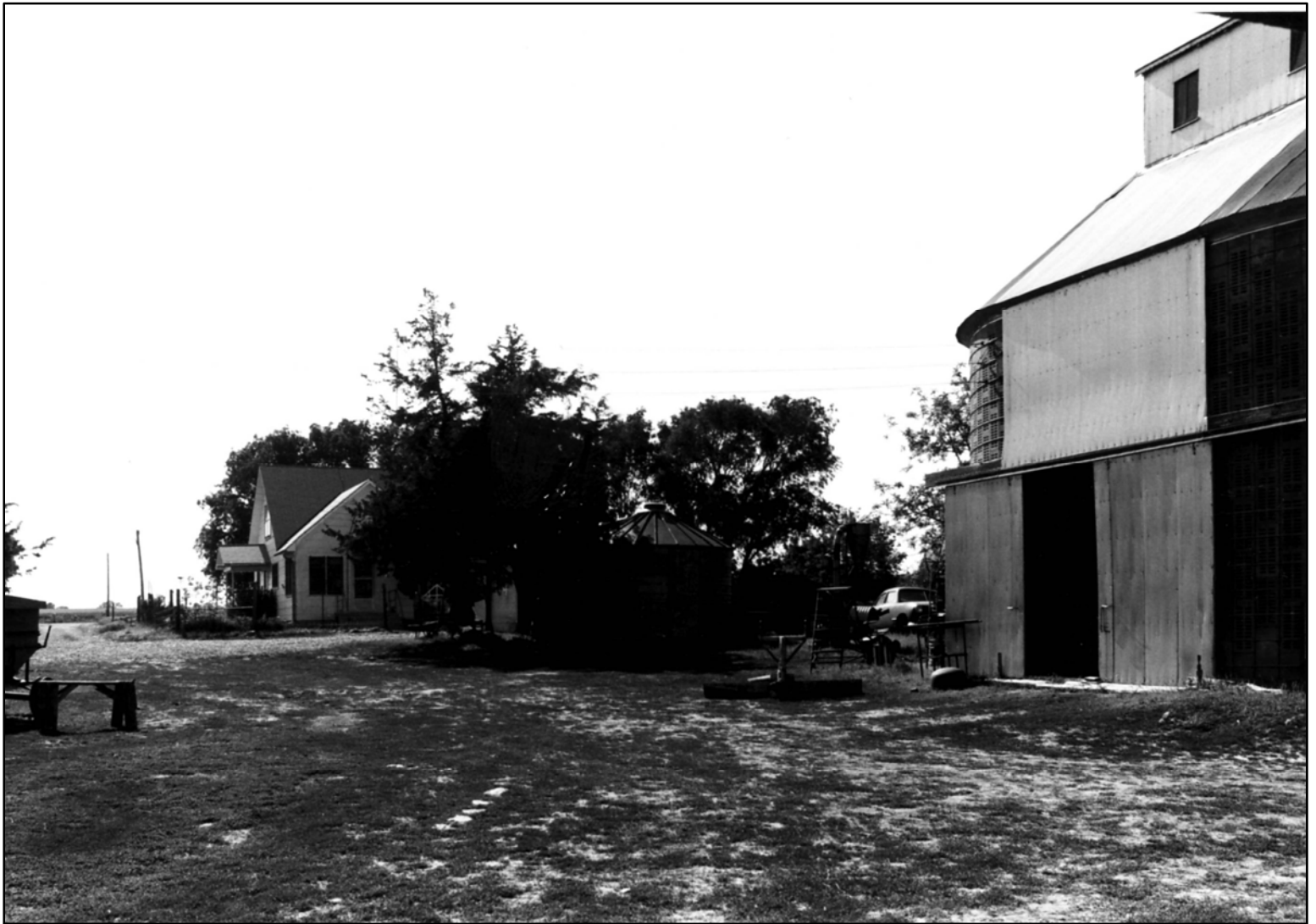
Photo 15 of 17 – view of farmstead looking northwest showing non-contributing 1950s farmhouse Photo by D. Murphy, Lincoln, NE, 1976 (DM 7606b:18)
