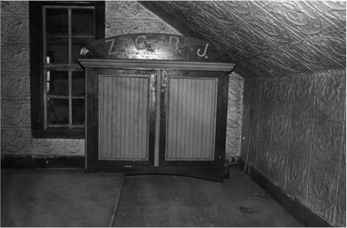
2nd floor, detail of robe closet, looking S Photo by John Carter, Oct 1980, NSHS (8010/1:26)
