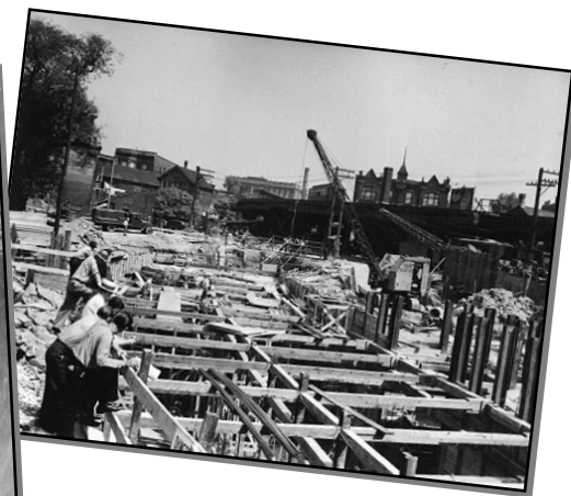
Employees of the Works Progress Administration building the Chicago subway system
