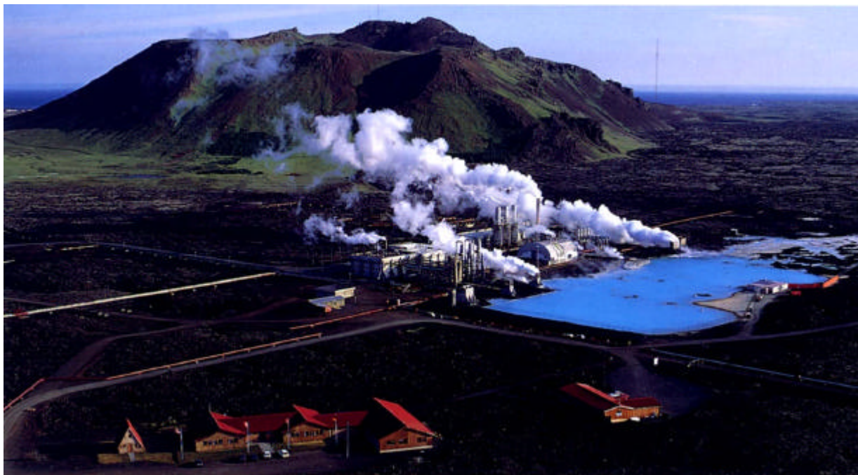
Figure 1. Svartsengi Power Plant aerial view.
