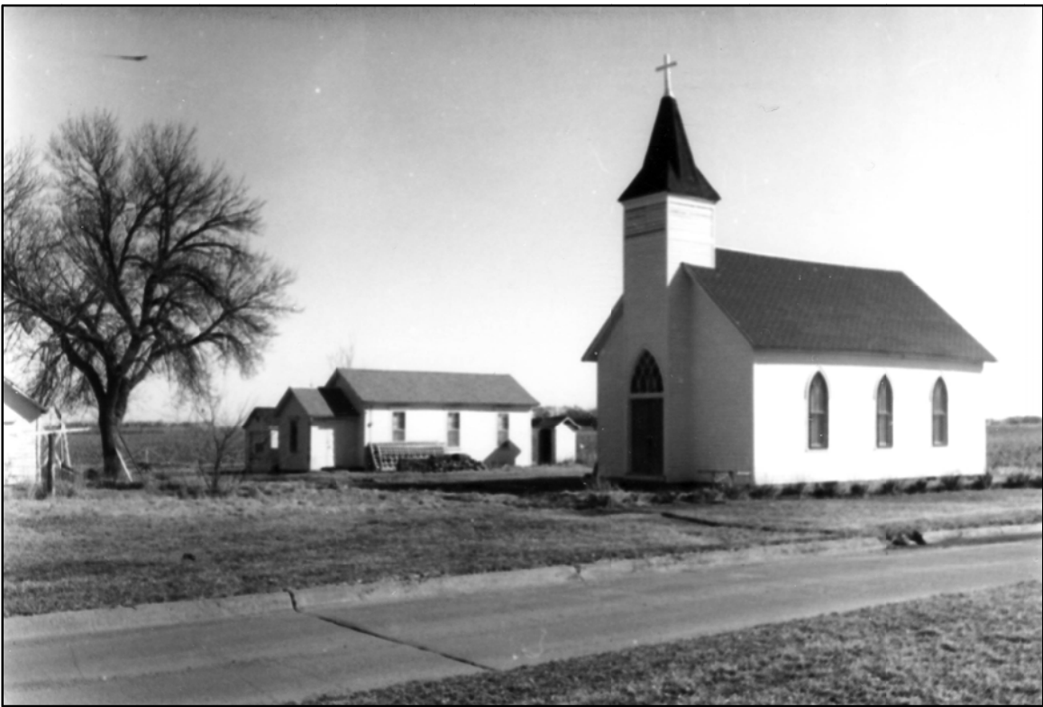
Photo 5 of 7 – outdoor museum looking east-southeast Photo by D. Murphy, 1976, NSHS (7602/1:36)
