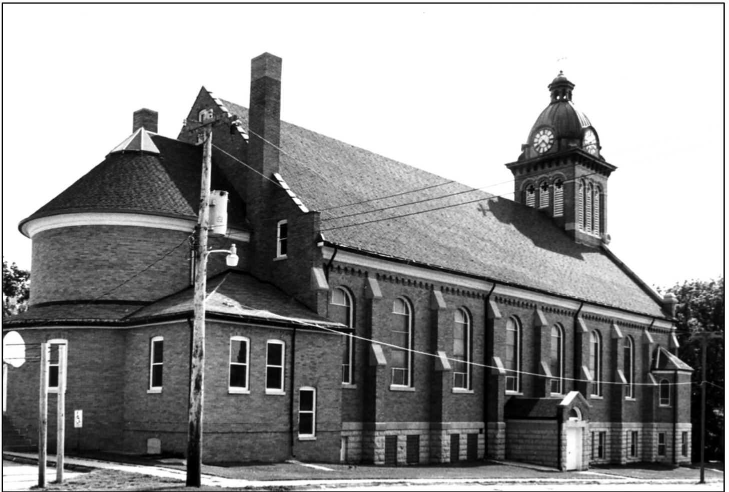
Aspect: NE – photo by Steve Pondelis, NSHS, June 1982 (8206/22:4)
