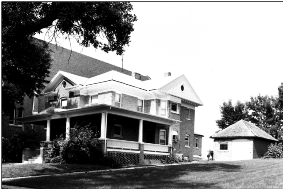
Rectory & garage, aspect: SW Photo by Steve Pondelis, June 1982, NSHS (8206/22:8)
