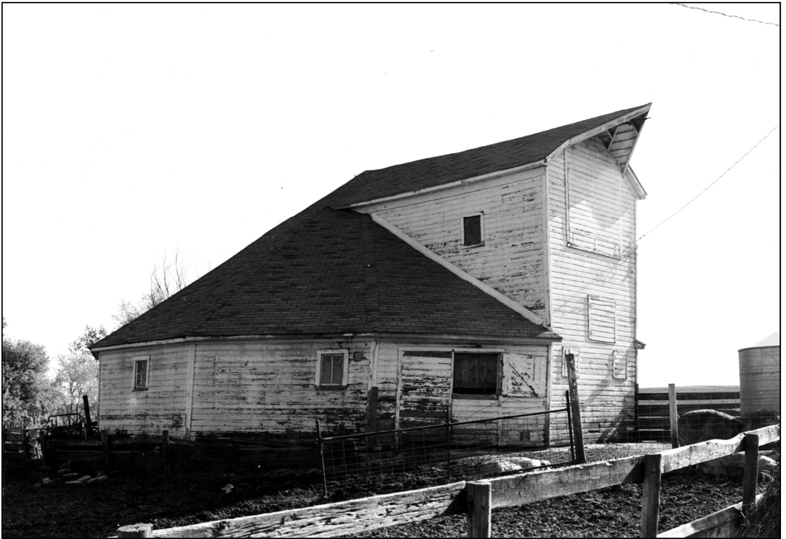
Photo 2 of 6 – view looking northeast showing south (front) and west facades Photo by Joni Gilkerson, May 1985, NSHS (8505/4:5)
