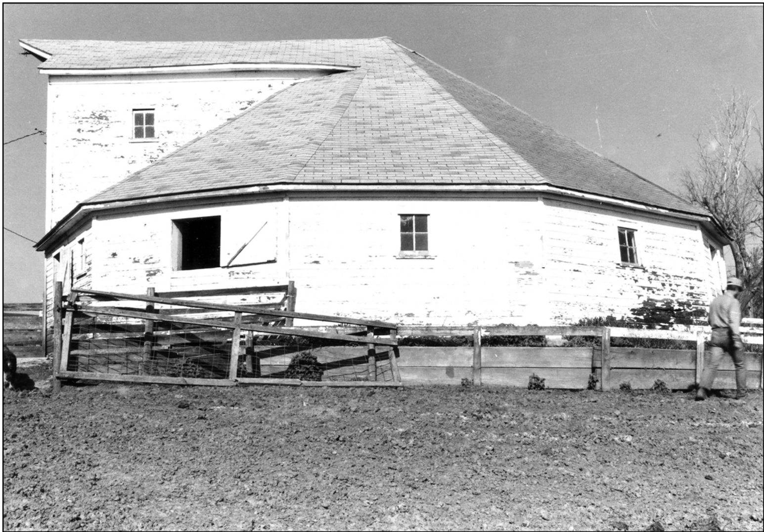
Photo 3 of 6 – view looking west showing east façade Photo by Janet Jeffries Spencer, May 1985, NSHS (8505/4:6)
