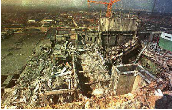
Chornobyl Reactor #4 as it looked before it was covered.
