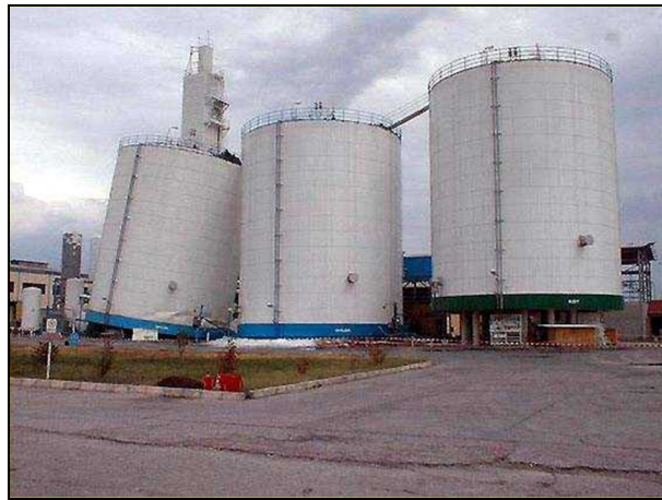
Figure 14. Elephant foot buckling of Tupras Refinery cylindrical tanks ( left ) and deformation of tanks in Kocaeli ( right ) after the 17 August 1999 Marmara Earthquake, Turkey.
