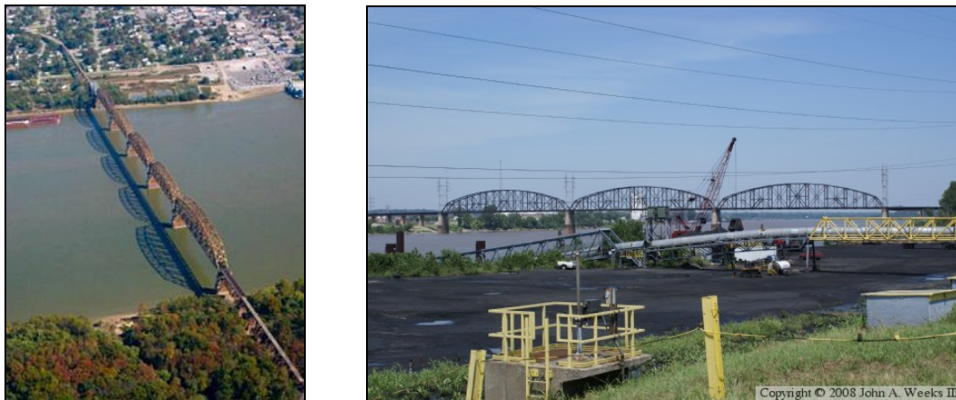
Figure 6. Metropolis Bridge, 1917 ( left ) and Menchants Bridge, 1889 ( right )
