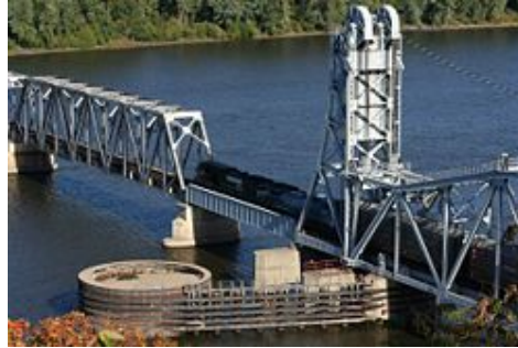
The Wabash Bridge looking southeast
