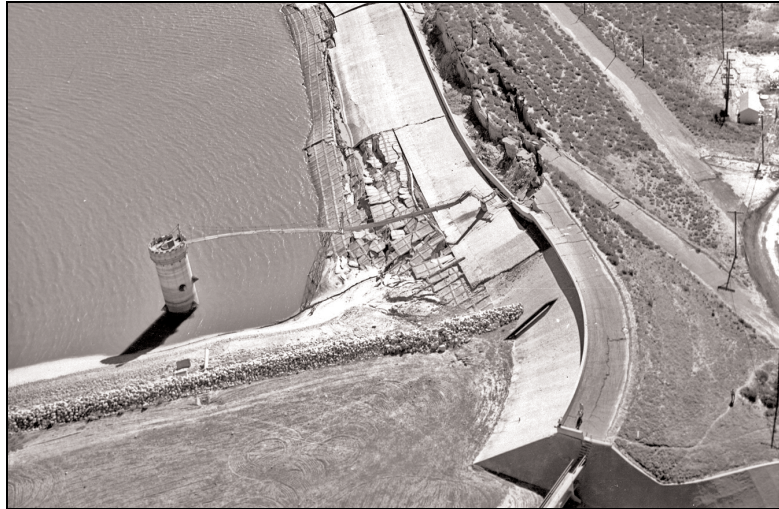
Figure 11. Damage at the Lower Van Norman Dam by the February 9, 1971, San Fernando, California, earthquake (FEMA, 2005).
