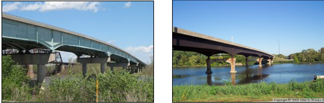
Figure 7. Lewis Bridge, 1979 ( left ) and Moline-Arsenal Bridge, 1982 ( right )
