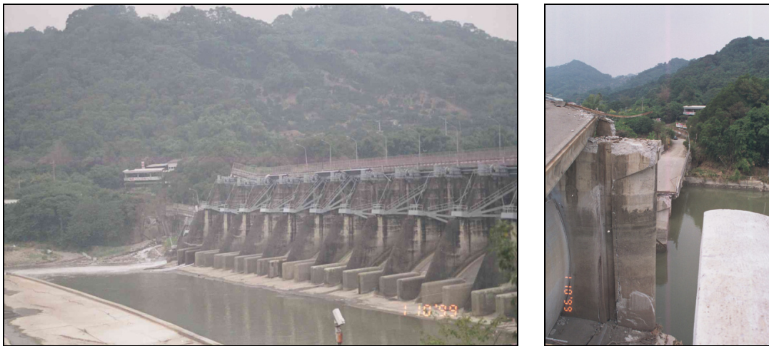
Figure 12. Dam suffered damage during the 7.6 magnitude 1999 Chi-Chi earthquake, Taiwan (Images by Prof. Y. Hashash, University of Illinois)
