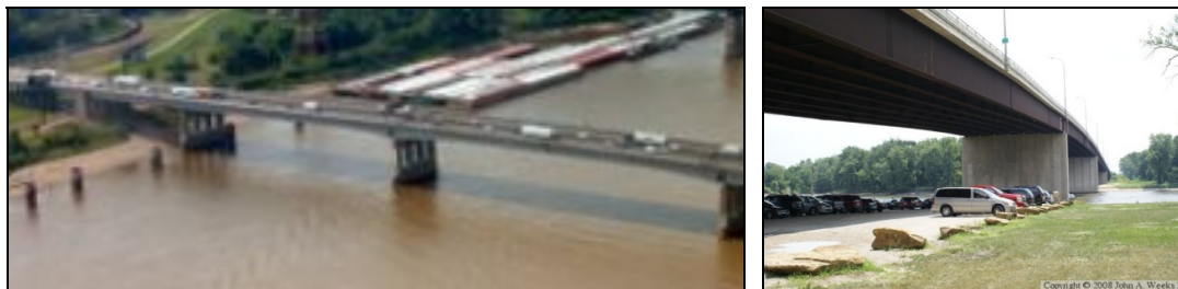
Figure 8. Poplar Street Bridge, 1967 ( left ) and Morris Bridge, 2002 ( right )
