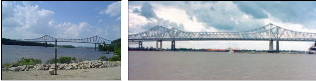
Figure 5. Savanna-Sabula Bridge, 1932 ( left ) and Crescent City Connection Bridge, 1988 ( right )
