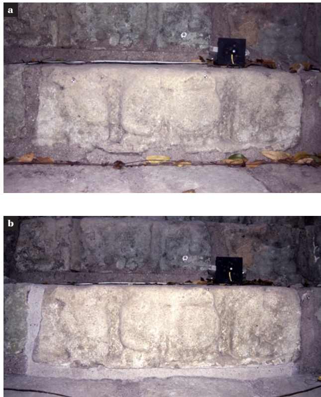
Figures 105a and b Treatment trial block 488, step 52, before (a) and after (b) mortar removal and repointing.
