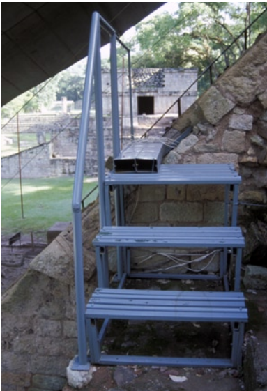
Figure 119 Access steps leading to a bridge across the south balustrade.
