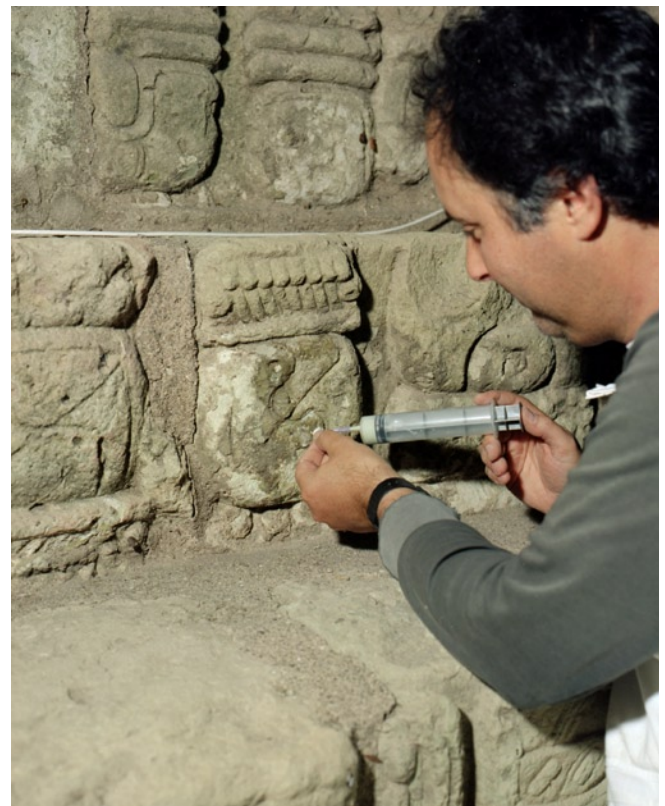
Figure 144 The microgrouting of a flaking surface of treatment trial block 578, step 61.
