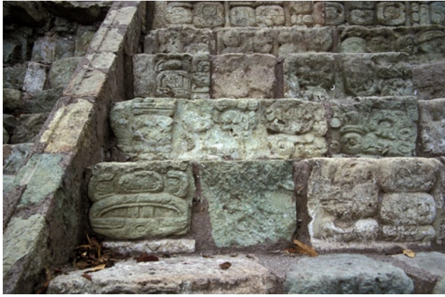
Figure 138 An old crack between the north balustrade and steps 54–58.
