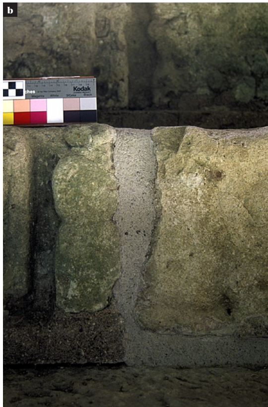
Figures 106a and b Comparison of two trial mortars for repointing: for block 406, step 43, the mortar was chosen to match the existing joint mortar (a); for block 488, step 52, the mortar was chosen to blend in with the variety of block colors (b).
