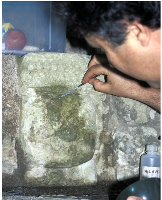
Figure 112 Edging flakes on block 578, step 61, with a lime-based mortar.
