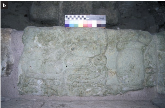
Figures 113a and b Treatment trial block 406, step 43, before (a) and after (b) treatment. There is an improvement in readability of surfaces after reduction of darkened consolidant from previous treatments and stabilization with edging repairs and with fills of lime-based mortars, colored with pigments to match the stone.
