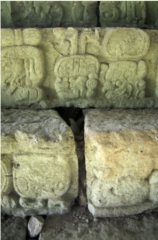
Figure 124 Area of mortar loss between blocks caused by burrowing animals.
