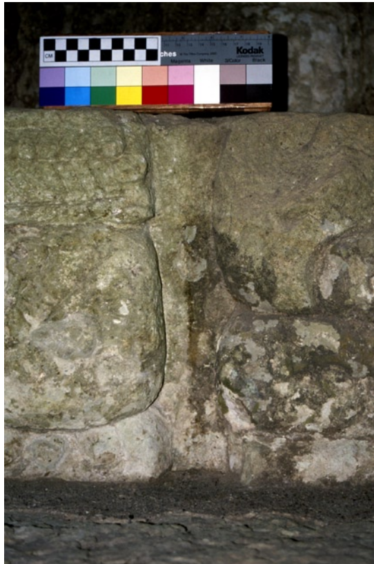
Figure 110 Stone surface shown after reduction of darkened consolidant (on the left); the procedure has not been performed on the right side.
