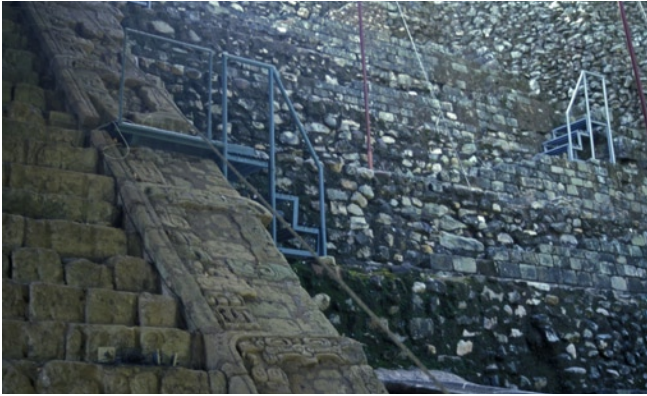
Figure 118 Current Stairway access across the south balustrade provided by steps at several points on the reconstructed terraces to the south of the Stairway, 2004.
