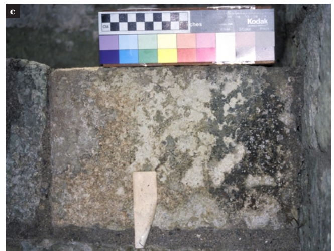
Figures 115a–c Uncarved block 68-2e, from the reconstructed upper steps, before treatment (a), after water cleaning of the left two-thirds (b), and eight months after the application by brush of Syton x-30 in distilled water (c) (left of tape, concentration 1:1; right of tape, 1:2).
