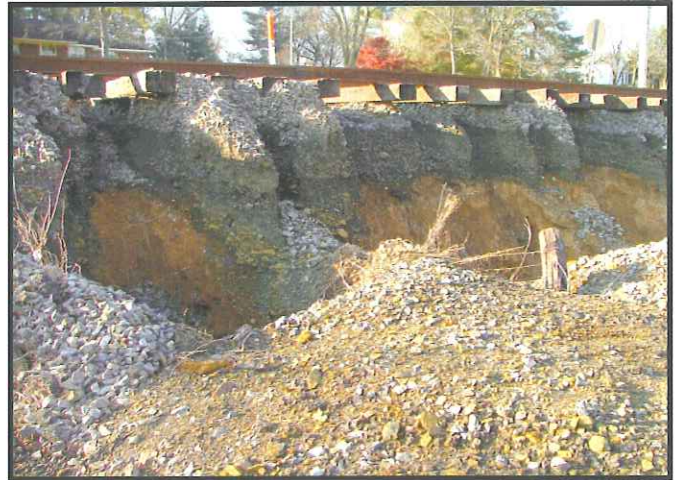
Even two months after the fact, substantial washouts are still apparent near LaFayette.
