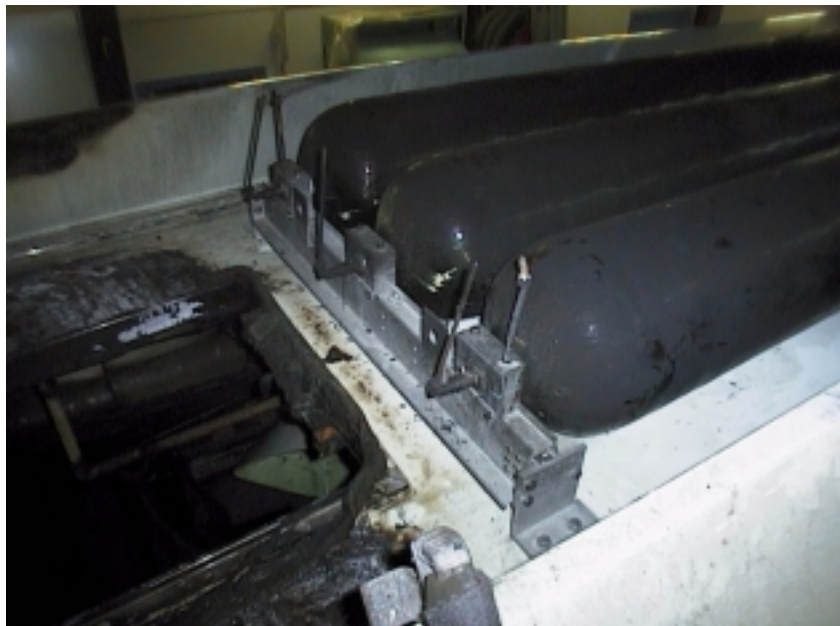
Fig. 28. Roof window and gas tanks.
