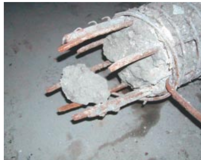
Figure 7.5b Ends of fractured reinforcing bars showing necking
