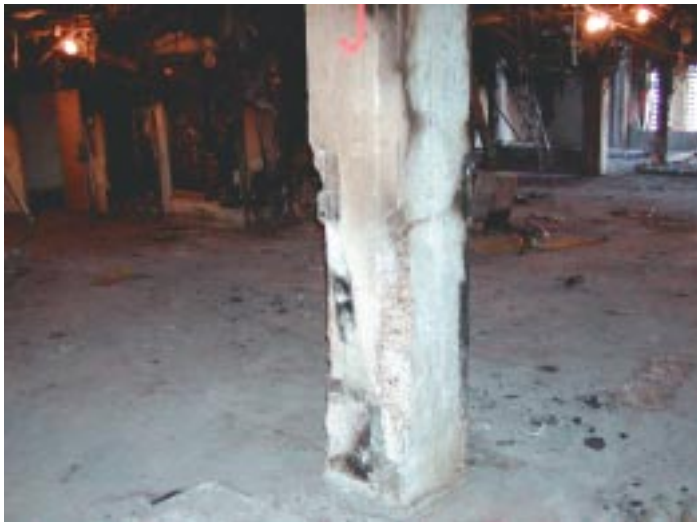
Figure 6.11 First-story column 7J
