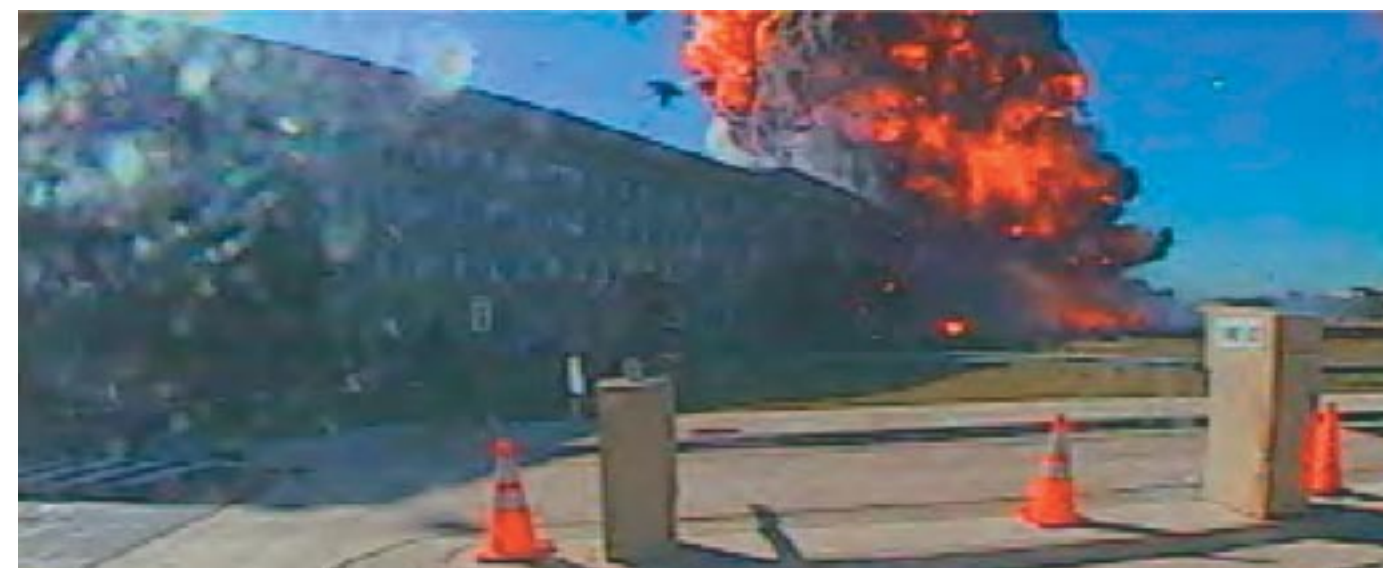
Figure 3.7 Fireball within four seconds of impact; the shadow of the smoke cloud visible on the ground provides a reference for determining the height of the aircraft.
