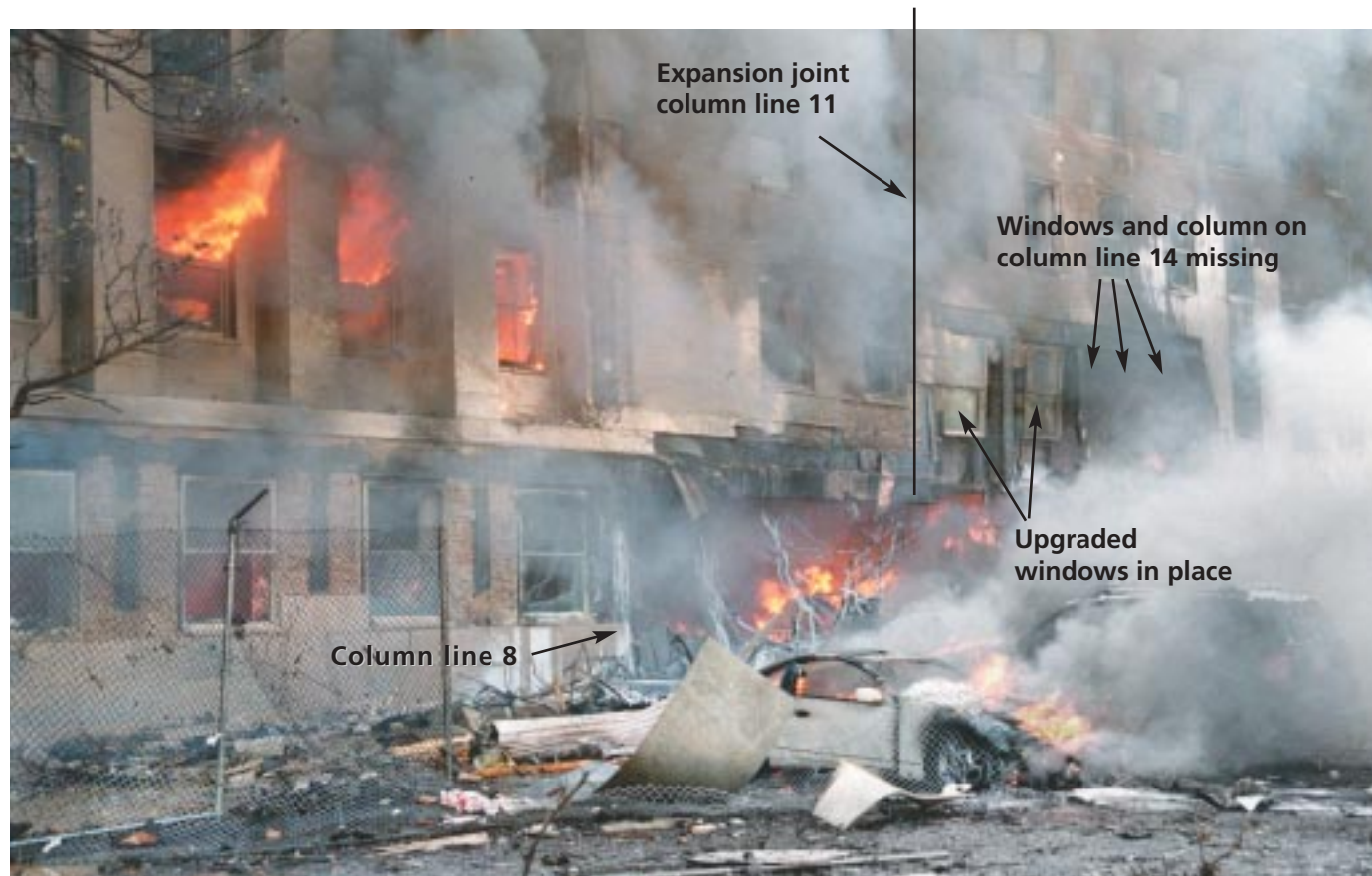
Figure 3.8 Northern portion of impact area before collapse
