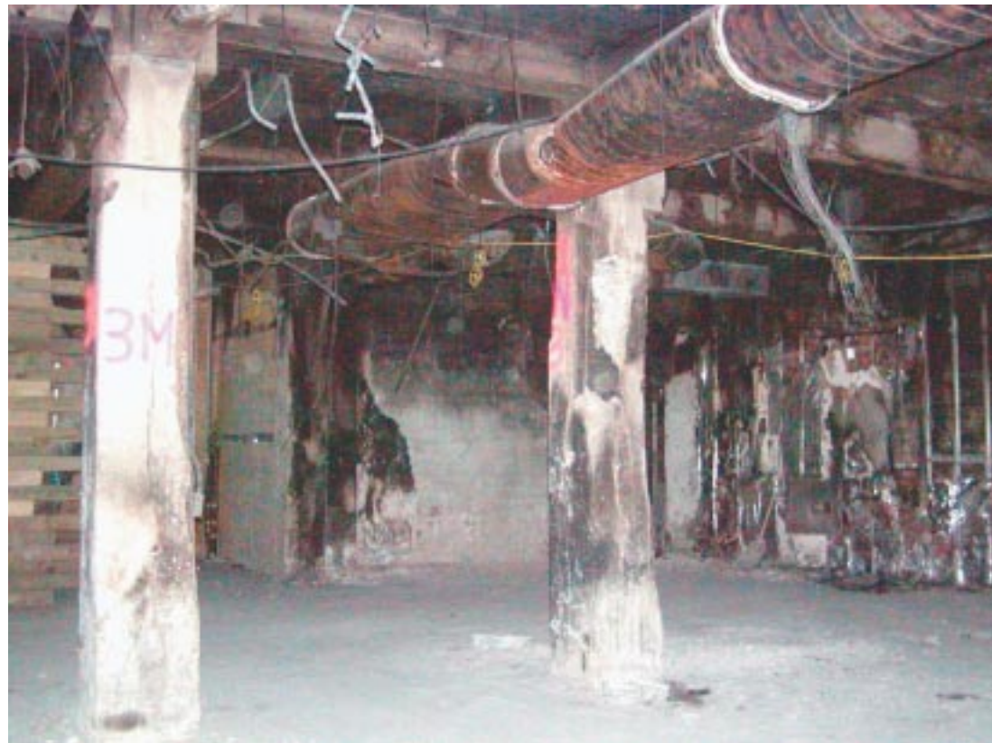
Figure 6.9 First-story columns 3M and 3N
