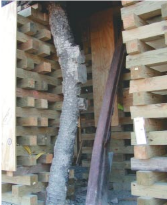
Figure 5.21 Column with triple curvature
