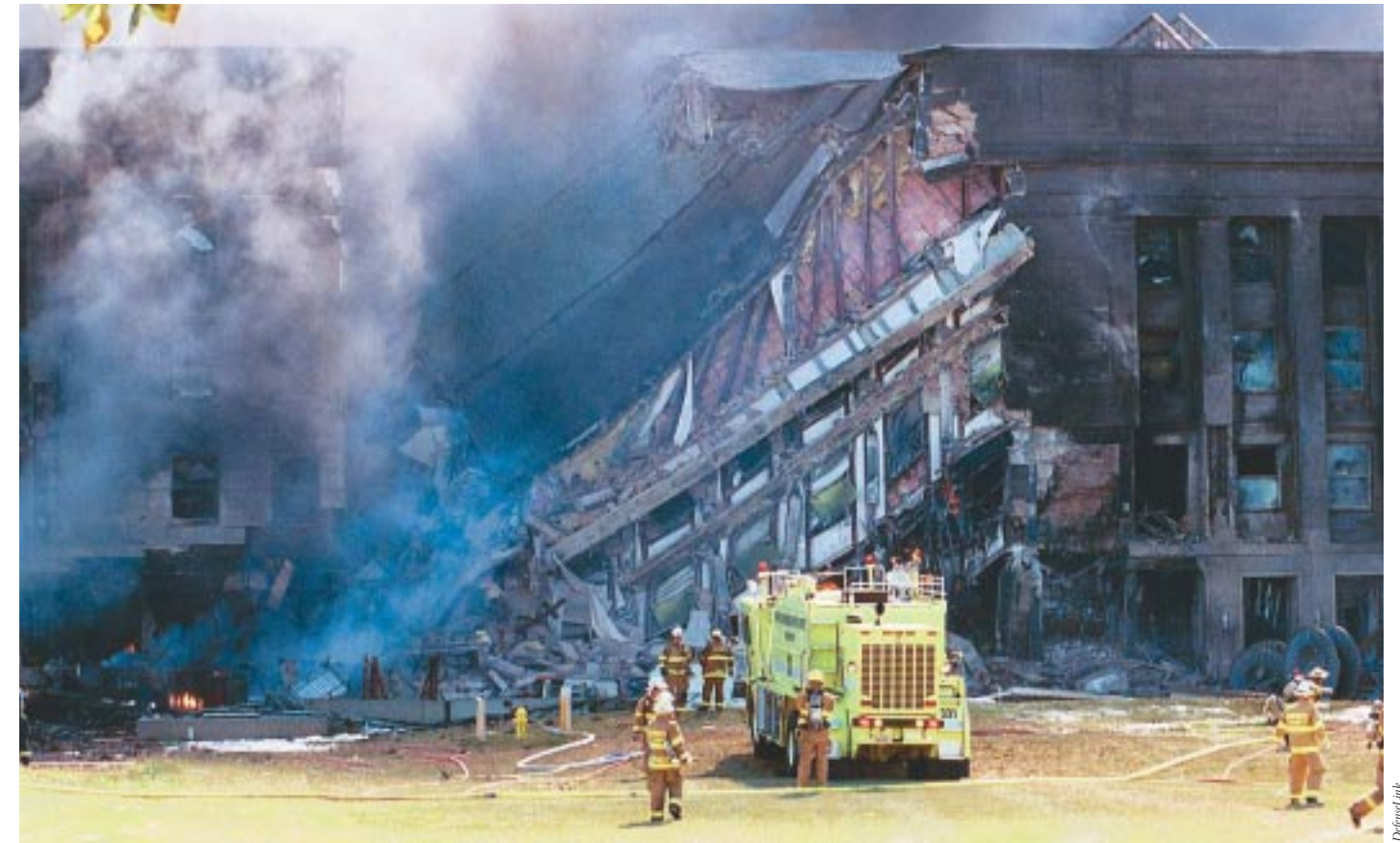
Figure 3.12 Ring E after collapse
