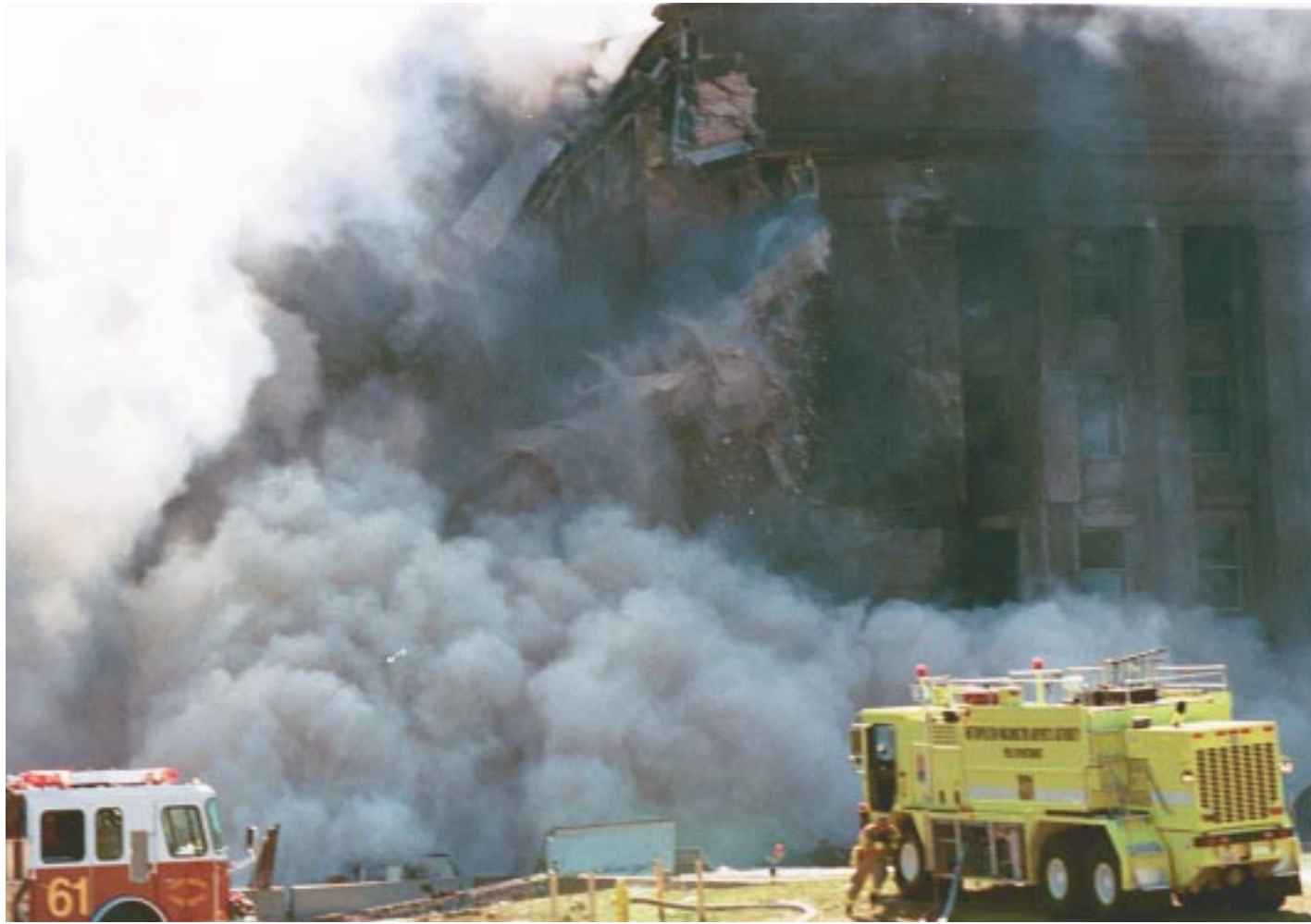
Figure 3.11 Portion of Ring E at moment of collapse
