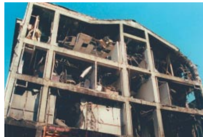
Figure 5.2 Beams and columns on north side of expansion joint
