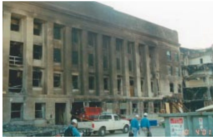
Figure 5.14 Upgraded windows in place
