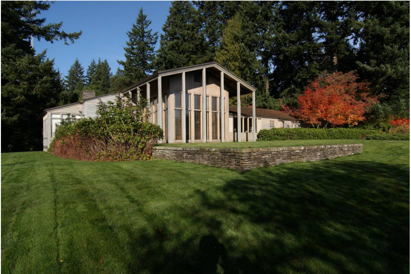
East elevation, looking northwest Jack Liu, photographer, October 2008
