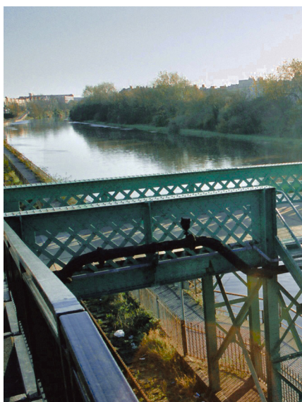
Vauxhall Bridge on the Cut at Southville
