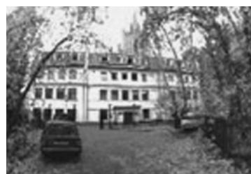
The newly reconstructed MCCME-IUM building
