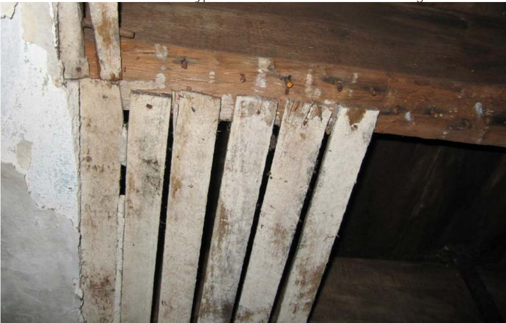
Image of circular sawn lath and nailing used in this area in the early 19 th century
