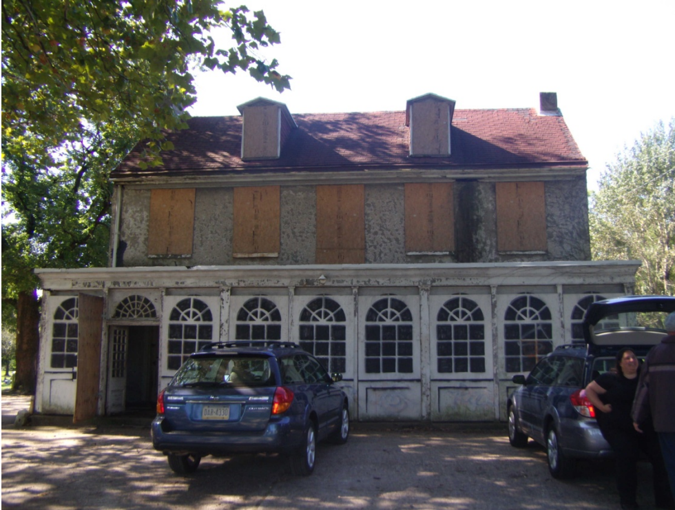
Front Elevation from October 2009
