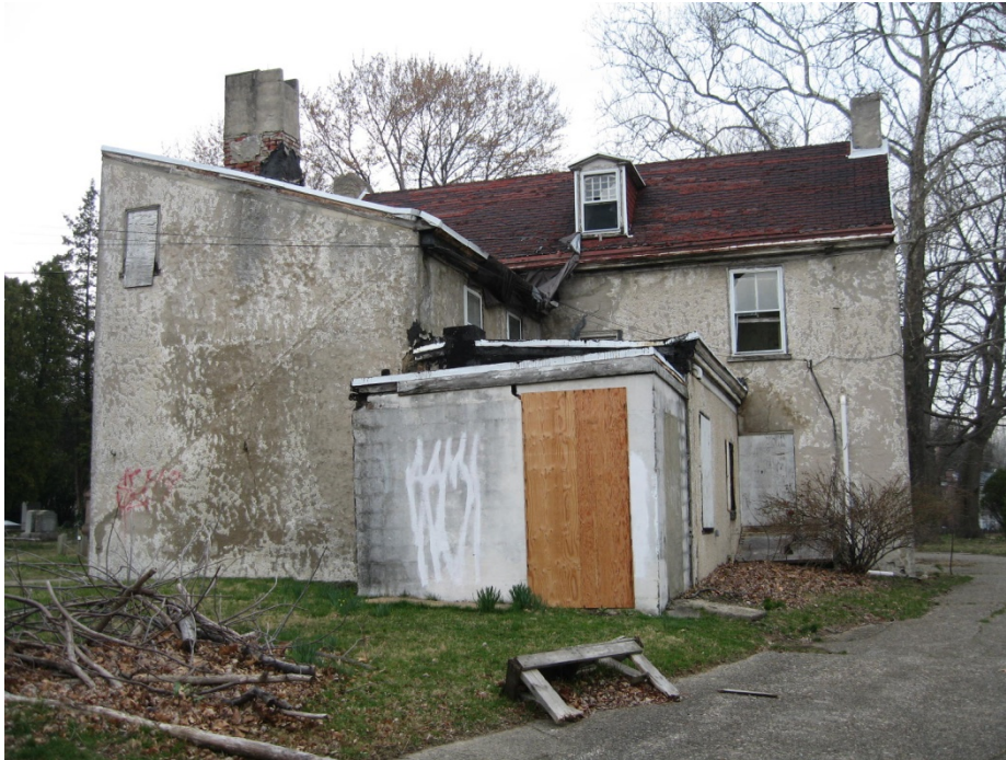
Rear View from March 2008
