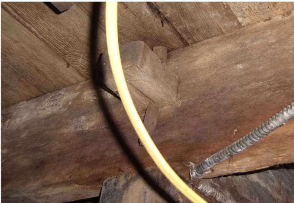
Image of tight mortise and tenon from the main house basement from July 2009
