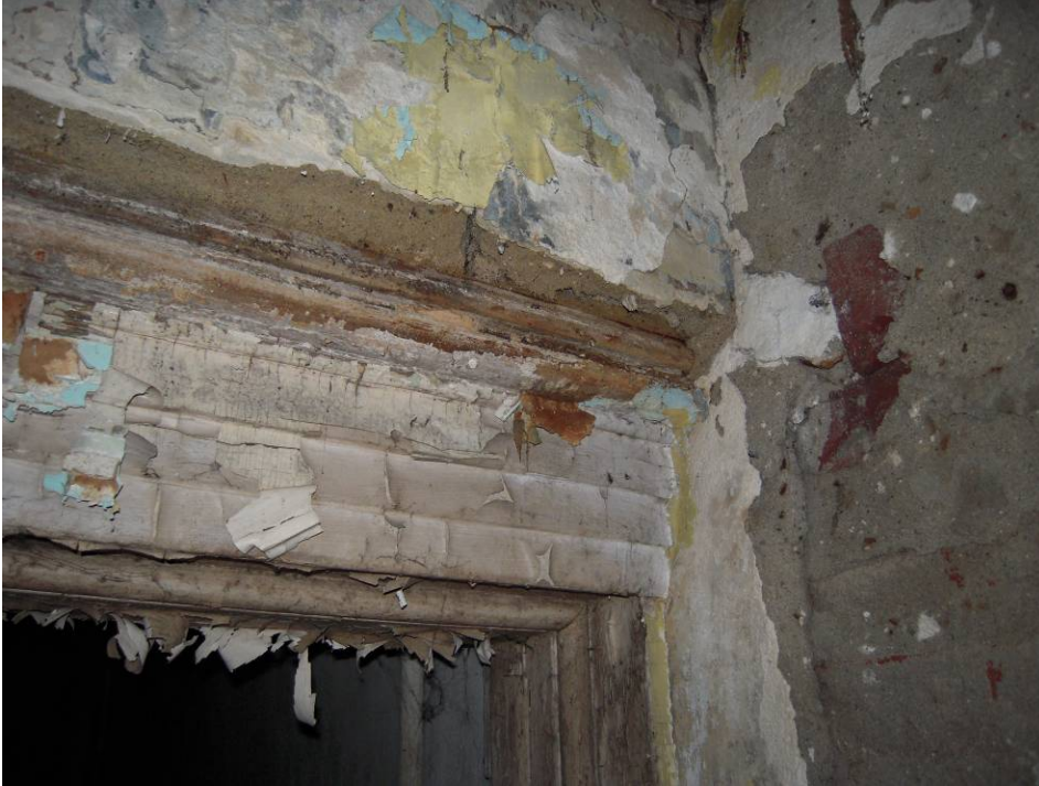
Stepped Cornice of Door Architrave, 1 st floor.
