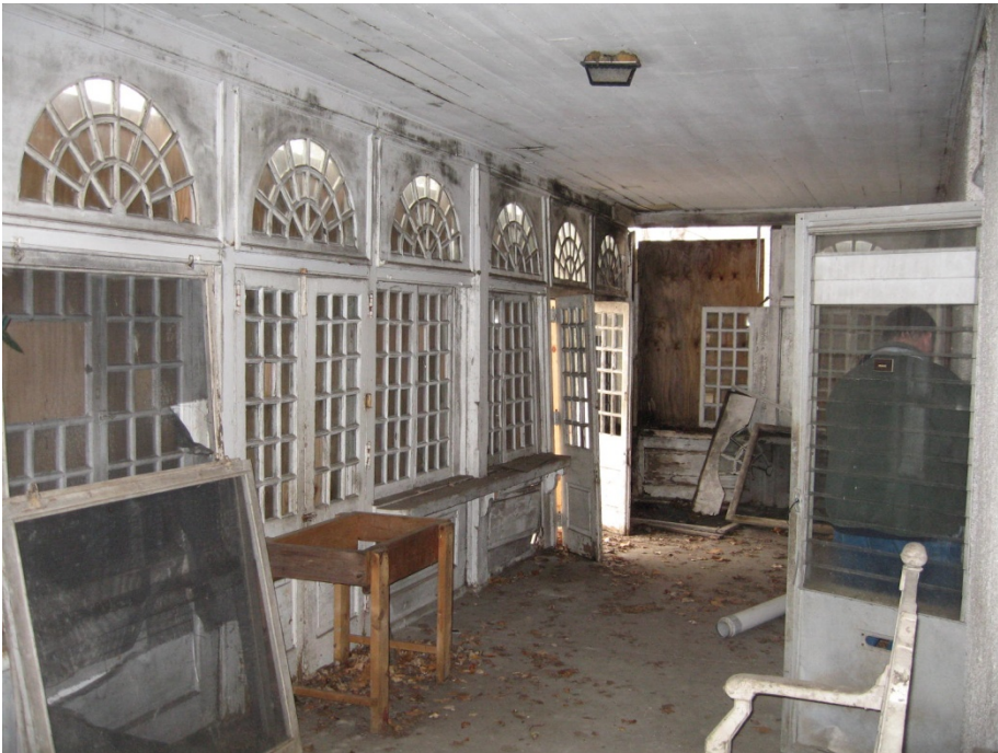
Image of porch interior from October 2009
