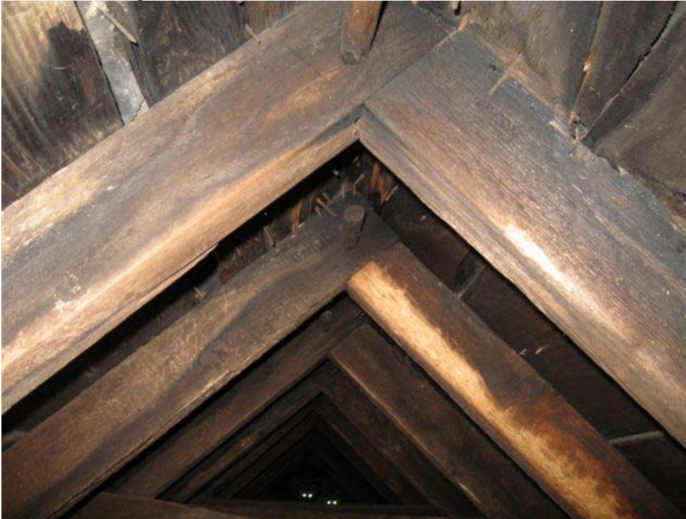
Image of the roof rafter framing from October 2009
