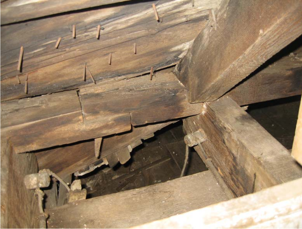
Image of the roof framing from October 2009
