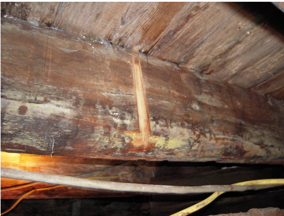
Area of sample GWCH01, ground level joist – near stairs.
