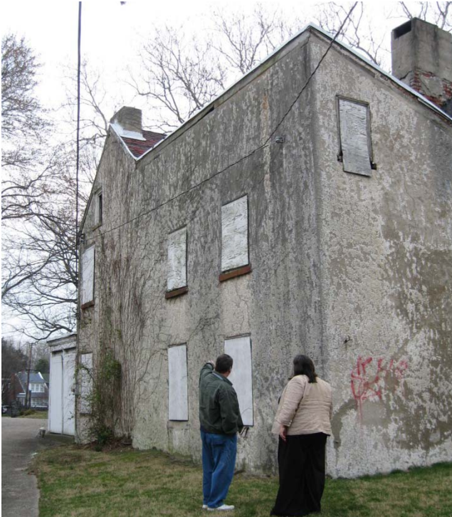
View of North façade of two story addition from March 2008
