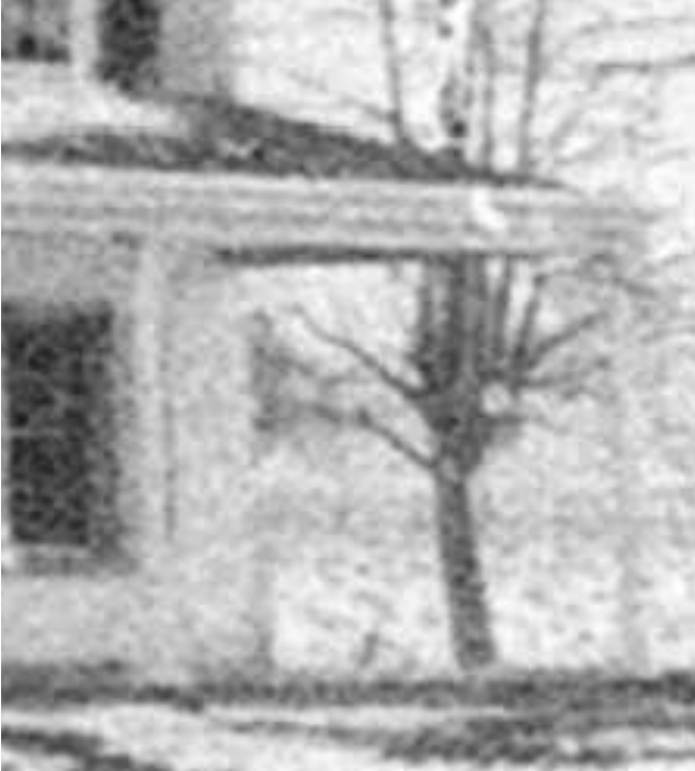
Image of edge of porch showing shadow at roof from near the Period of Significance (1830 - 1850)
