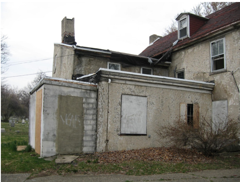
Rear View from March 2008
