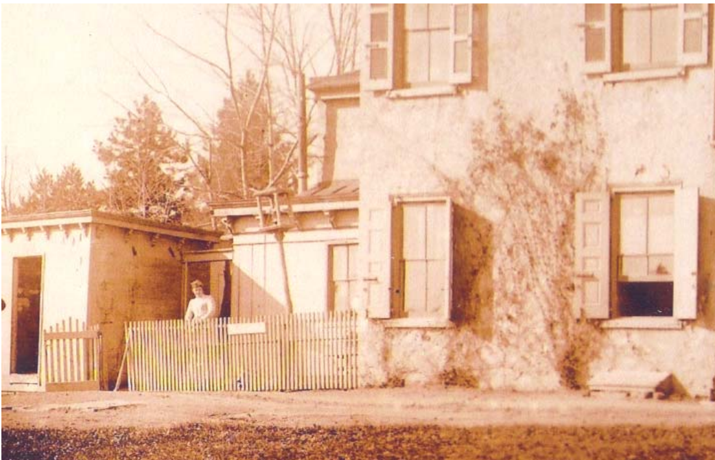
View of the additions on the house in the early 1900's: note the metal roof and window locations on the single story addition.
