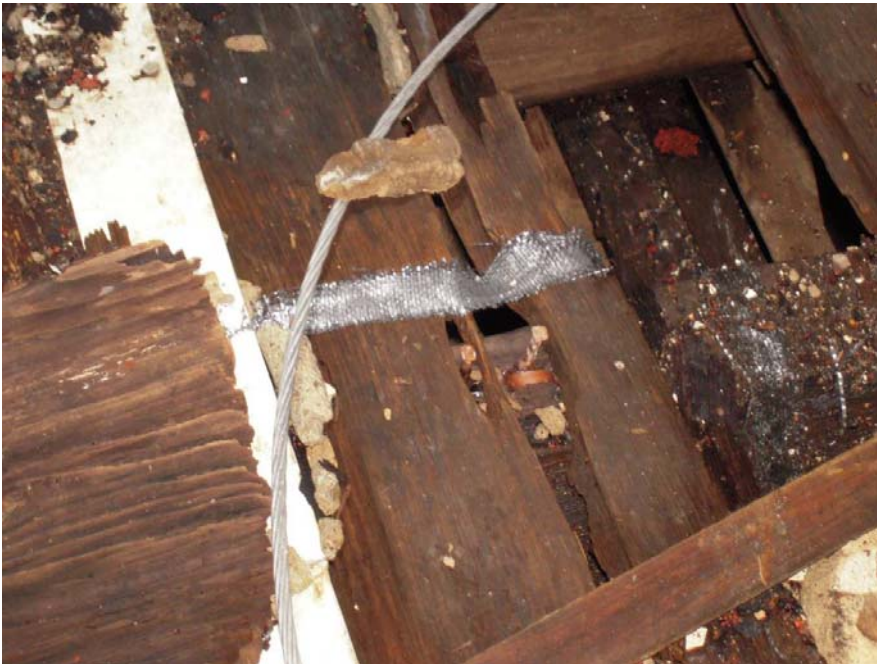
Area of wood flooring, 2 nd Floor, with 19 th century evidence
