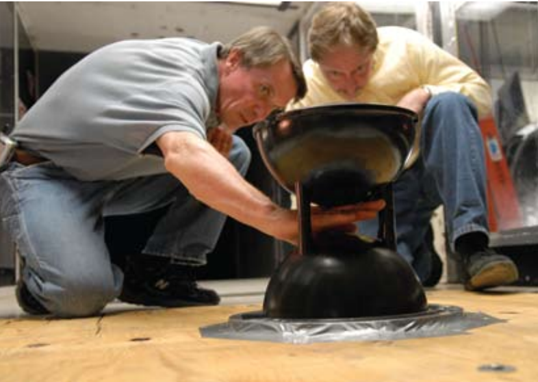
Tech alumnus Pat Johnson and Jim Jones, associate professor of architecture, inspect the installation of the V2T roof vent prototype in the Virginia Tech stability wind tunnel.
