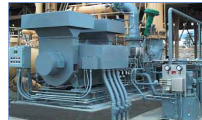
GE recently modified an axial turbine at a geothermal facility in the western US to a radial turboexpander.
