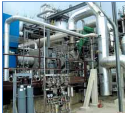
Located in Sicily, Italy, an Integrated Gasification Combined Cycle facility uses a GE Turboexpander-Generator to reduce the fuel gas pressure into its gas turbines. At the same time it produces 10-MW of electricity by expanding 313 MMSCFD (350,000 Nm 3 /hr).
