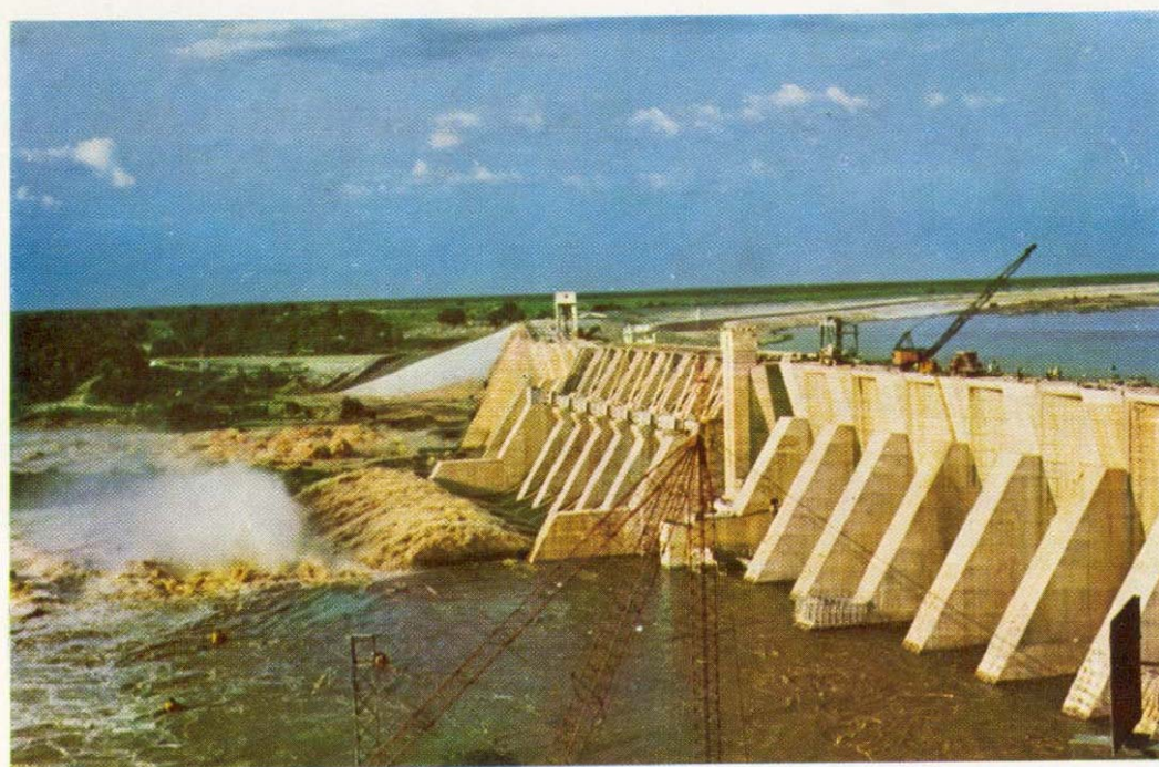
Figure 2-5 Roseires dam passing flood water in July 1966.
