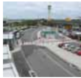
Brisbane Airport, Queensland, Australia
