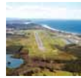
Gold Coast Airport, Queensland, Australia
