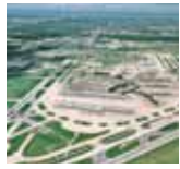
Chicago O'Hare International Airport, Chicago, IL, U.S.A.
