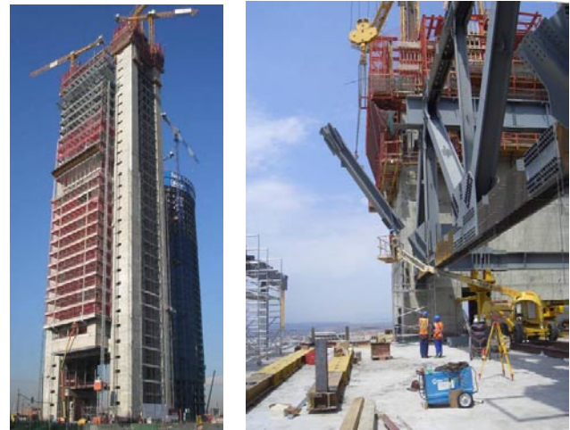
Figure 6. Caja Madrid Under Construction (Halvorson and Partners, 2007)
