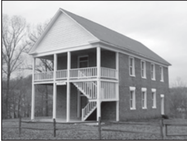
This school building built in 1901 was used as the home for Maxwell Academy and then later as a public school before it was closed in 1942.
