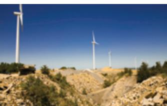
Eight of the project's 23 wind turbines sit atop a rehabilitated surface mine. To encourage the productive use of this land, the Pennsylvania Energy Development Authority supported the Casselman project with a \$500,000 grant to offset increased development costs. In addition, the former mining site will also host the wind farm's operation center, collector transformer and interconnection facility.
