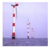
The near-shore wind turbine park, Lely, owned by Energie Noord West, consists of four NedWind40 turbines with a combined power of 2MW.
