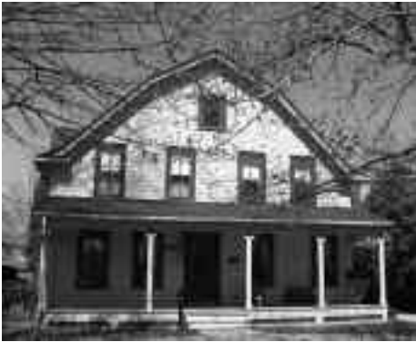
Backman House 1894 Grocery Store and Home 194 Moross Road
