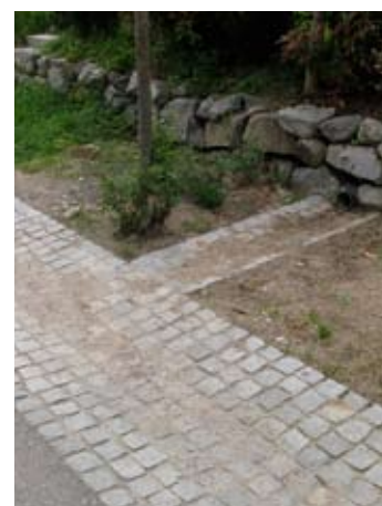
Permeable drainage channel
