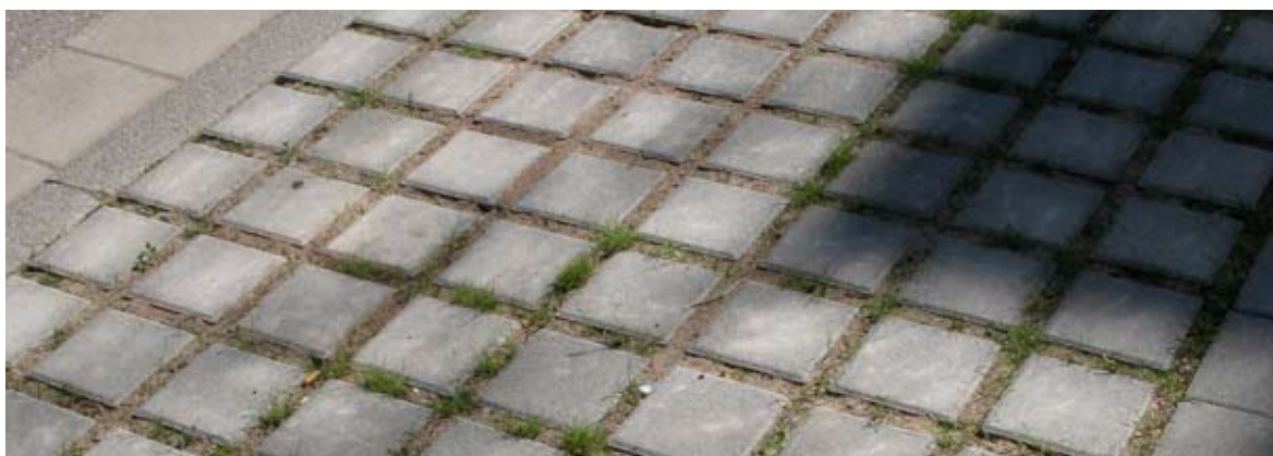
Permeable paving detail
