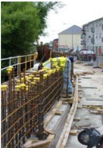
Construction of flood protection wall and demountable barriers in Clonmel
