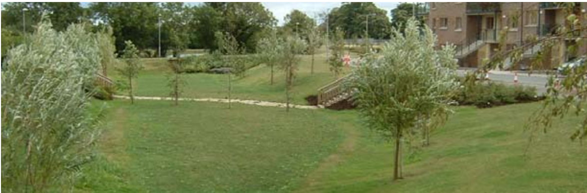
Detention basin and public open space, Carrickmines, Dublin
