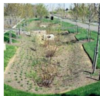
Bioretention device used as part of a Sustainable Drainage System
